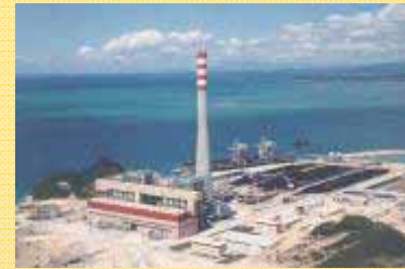
2 x 367.5 MW Pagbilao Power Plant, the Philippines
