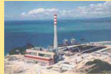
2 x 367.5 MW Pagbilao Power Plant, the Philippines
