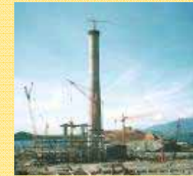
2 x 600 MW Sual Power Plant, the Philippines
