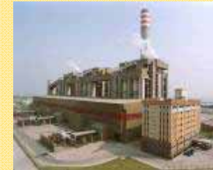
3 x 660 MW Shajiao C Power Plant, China
