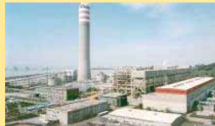
2 x 350 MW Shajiao B Power Plant, China
