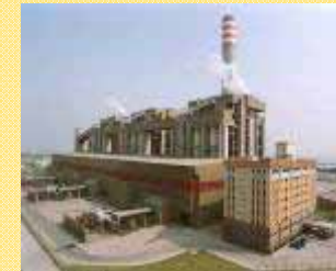
3 x 660 MW Shajiao C Power Plant, China
