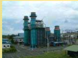
135 MW Sengkang CCGT Power Plant, Indonesia
