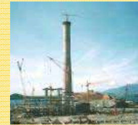
2 x 600 MW Sual Power Plant, the Philippines
