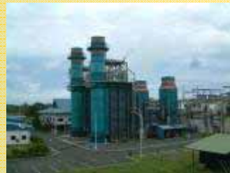
135 MW Sengkang CCGT Power Plant, Indonesia
