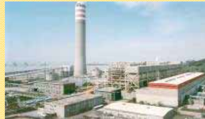
2 x 350 MW Shajiao B Power Plant, China
