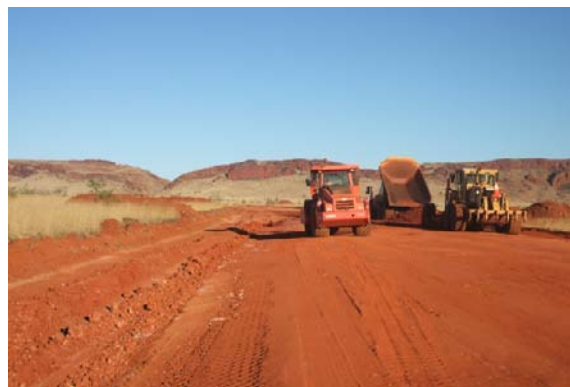
Haulage road works at Spinifex Ridge – June 2010
