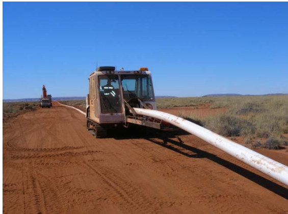
Water pipeline construction to the De-Grey borefield – June 2010
