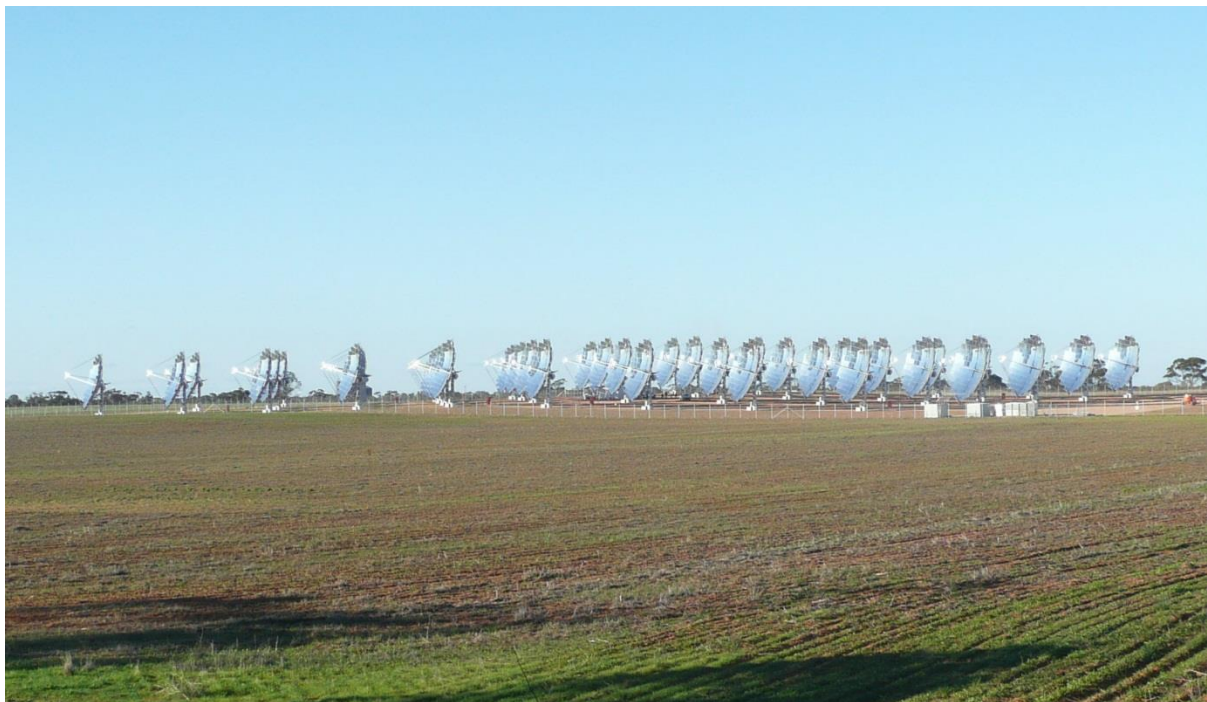
Above: the completed Mildura ‘Dense Array’ CPV Demonstration Facility, June 2013
