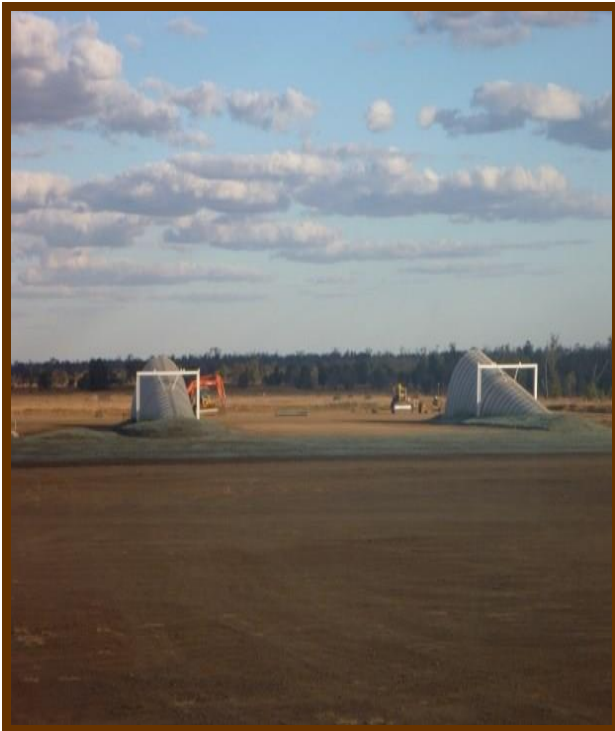
Figure 1 : Portal arches at Eagle Downs
