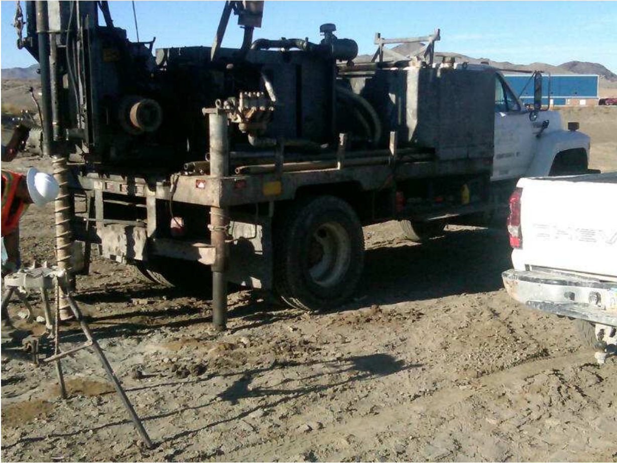
Figure 1: Auger drilling on site
