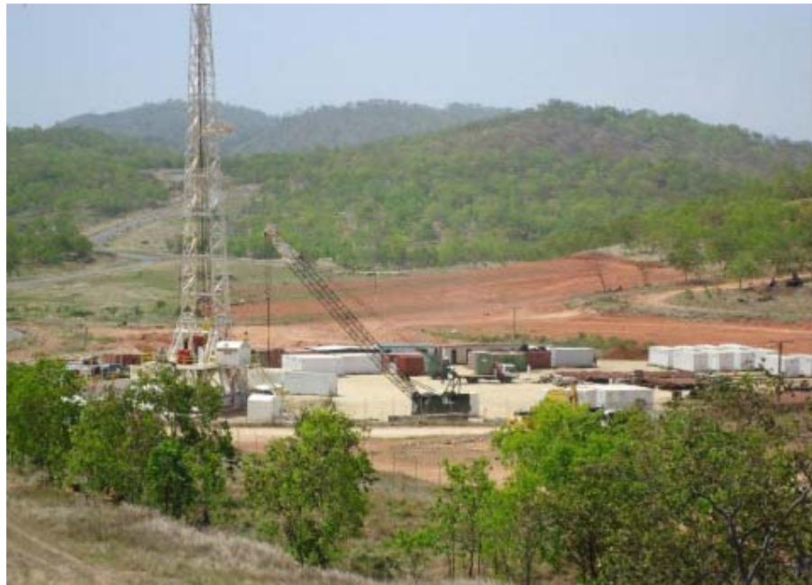
Figure 3 - Western Drilling Rig and Laydown Area
