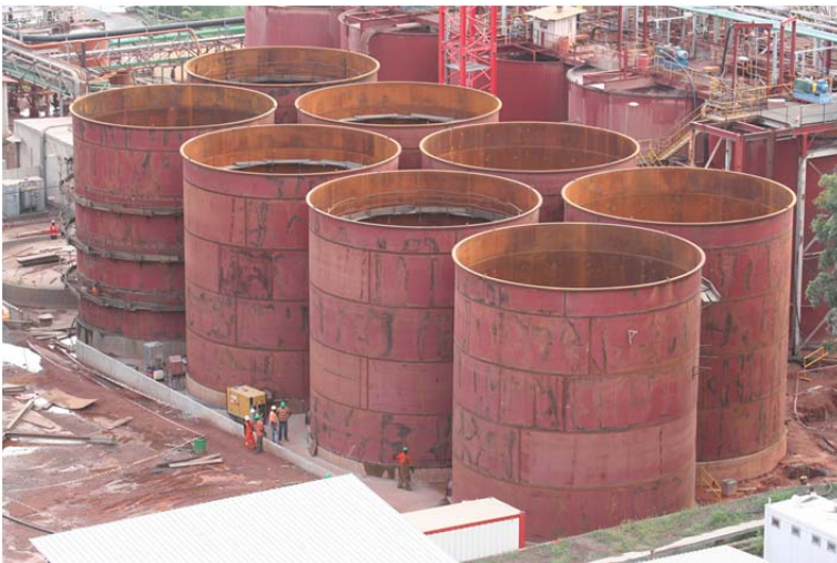
Figure 2. Oxide CIL tank erection October 2013
