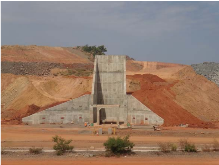
Figure 1. Completed Oxide crusher structure - October 2013
