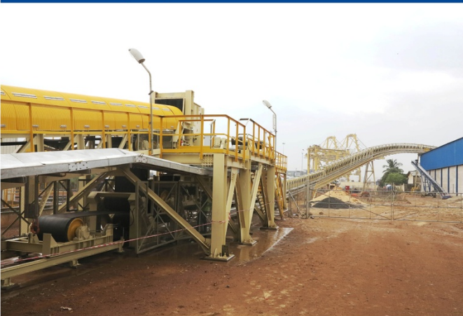
Conveyor system at port
