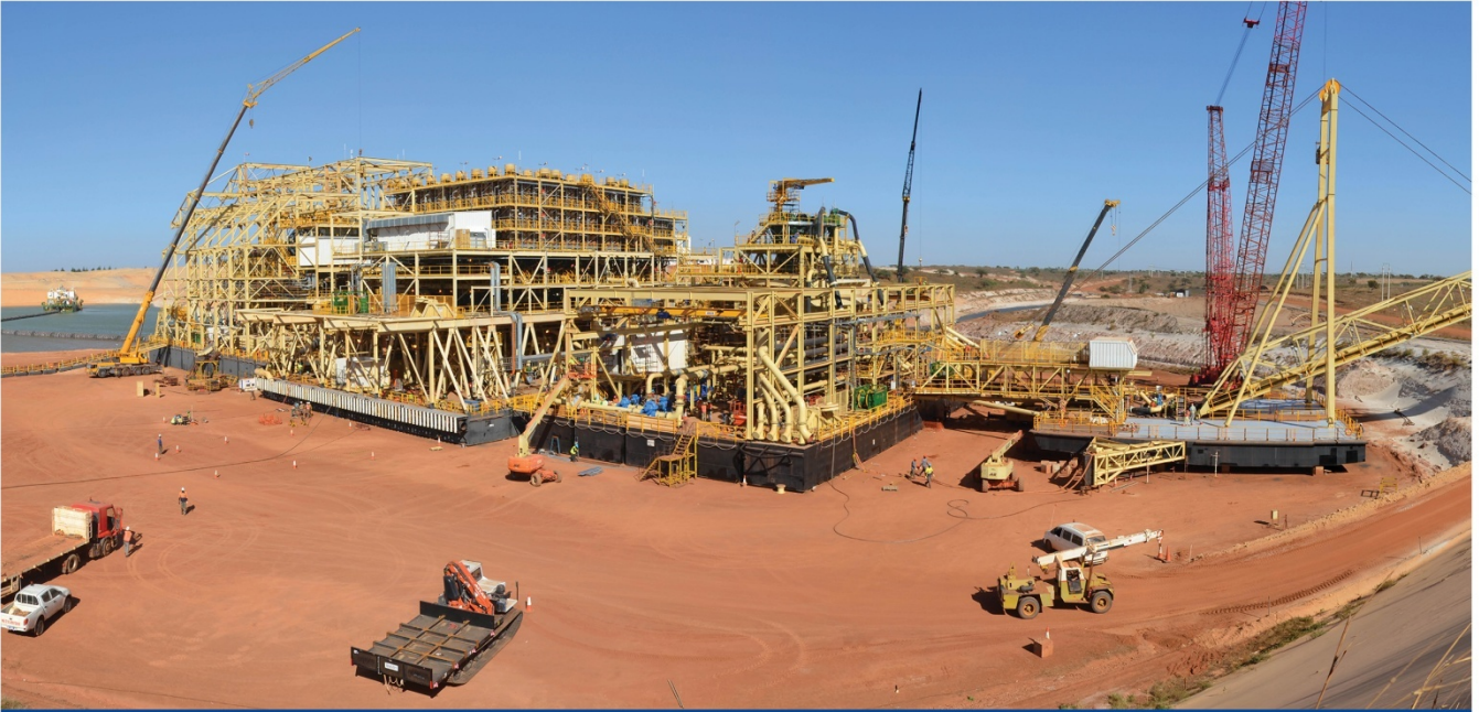
Dredge and Wet Concentrator Plant (WCP)
