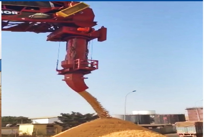
Commissioning conveyor / loading system with sand
