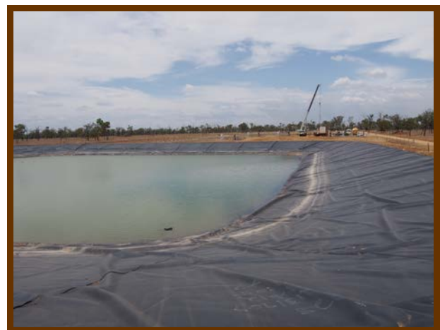
Figure 1 : Raw water dam at Eagle Downs
