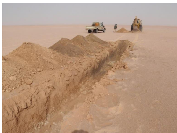
Fig. 4: Trench showing desert terrain, and white calcrete mineralisation
