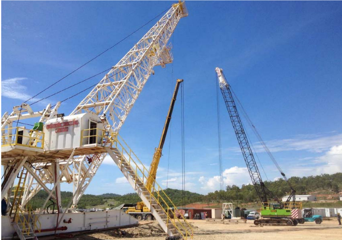
Figure 3. Western Drilling Rig during rigging down operations in December 2013.
