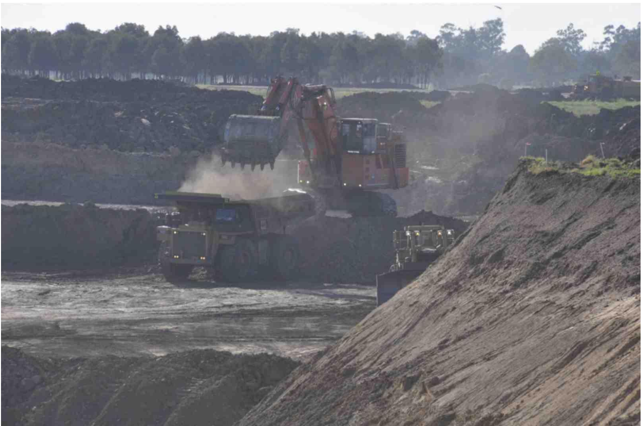
Figure 1 - Pre-stripping at Baralaba North
