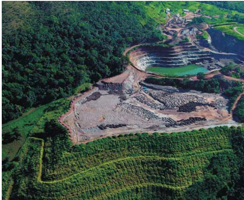
Figure 2. Sertão circa 2005. Note that the plant and equipment visible at the top (NE) of the photo does not remain on site, and does not form part of the transaction.
