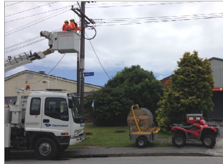
First aerial deployment began in Greymouth in December in association with local lines company.
