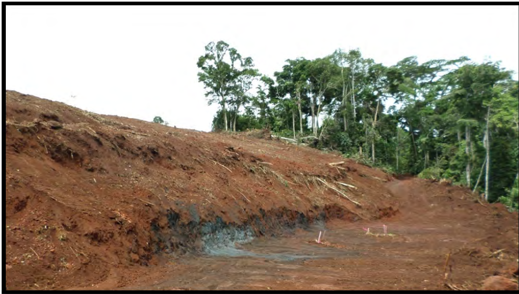
Figure 3 – Initial Earthworks at the Nabeba Trial Mining Area
