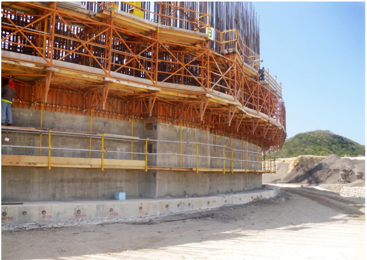
First Concrete Stage Slipform of LNG Tank Completed
