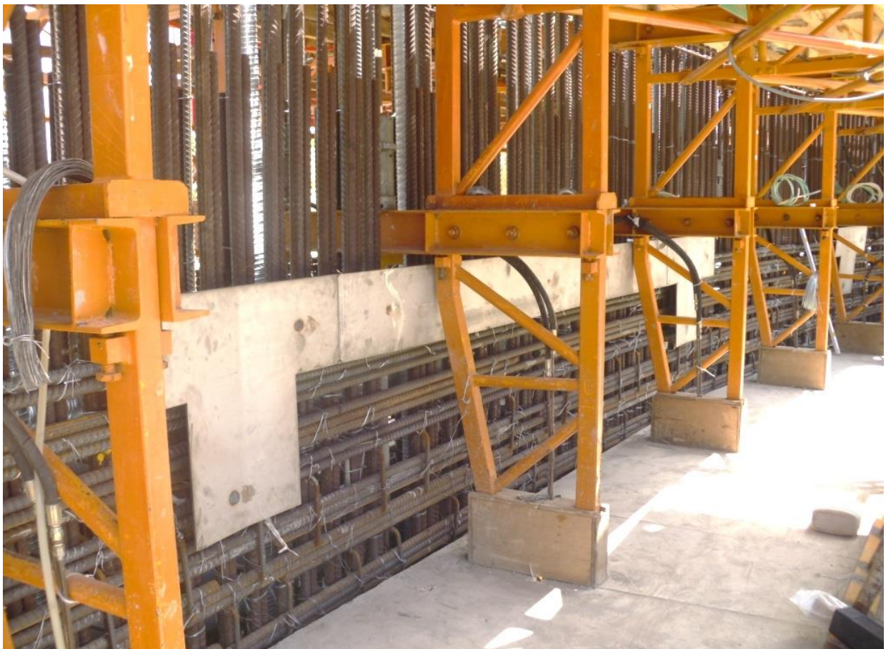
Stainless Steel Embedment Installation
