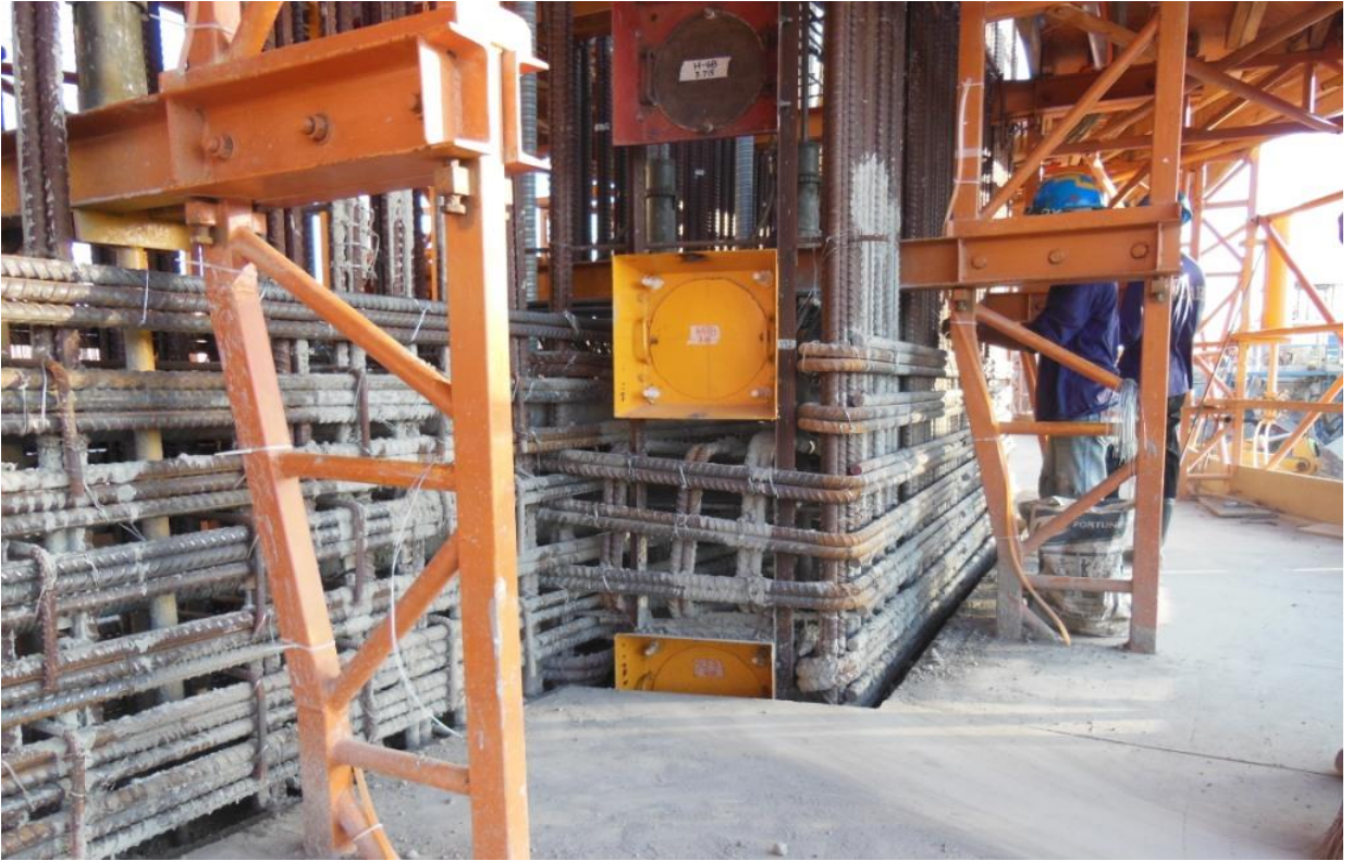
Reinforcement & Boxout Anchorages for Post Tensioning for LNG Tank
