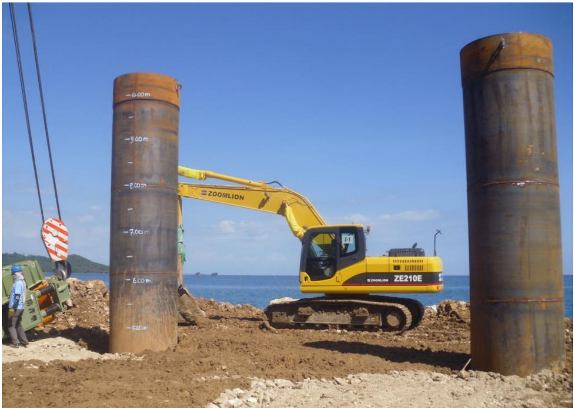
Marine Works & Jetty Piling
