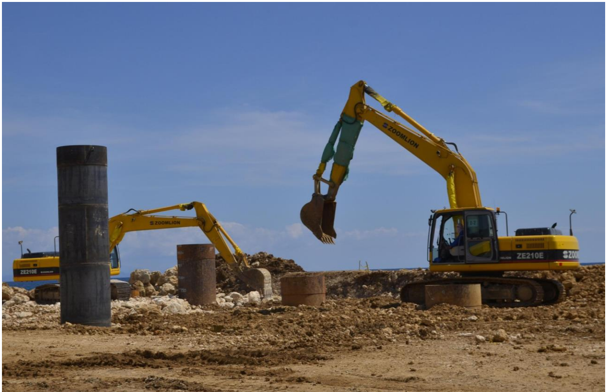
Grading, Leveling and Installation of Bored Piles
