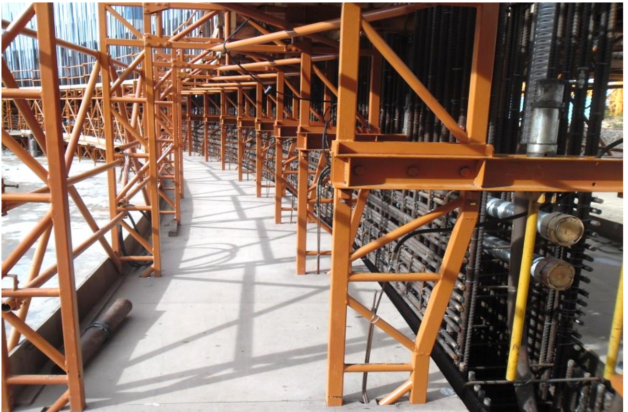
Slipform Working Deck Completed for LNG Tank
