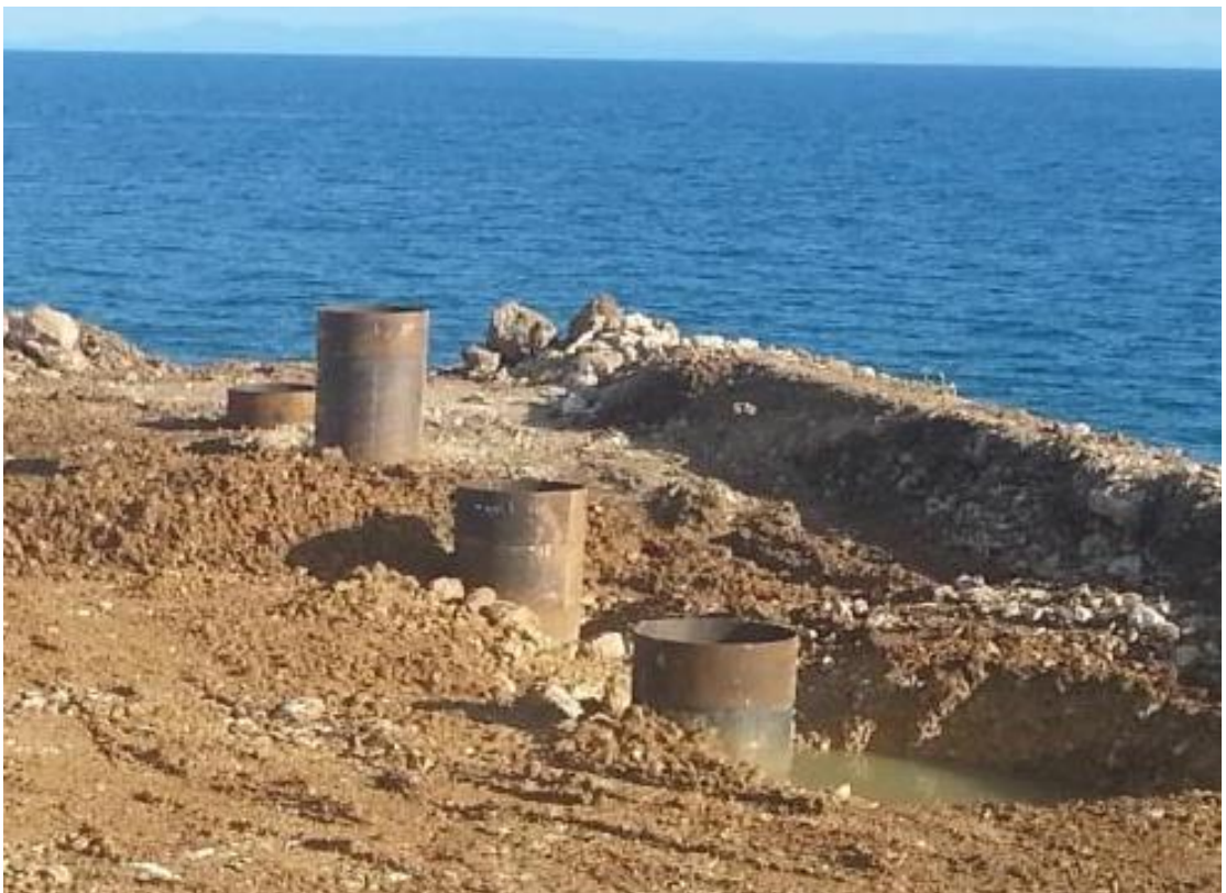
Marine Works & Jetty Piling
