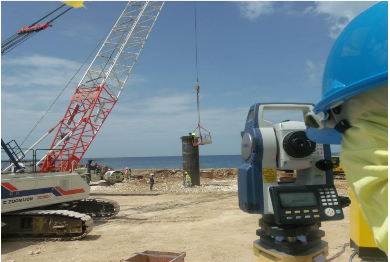
Checking the alignment of LP-6
