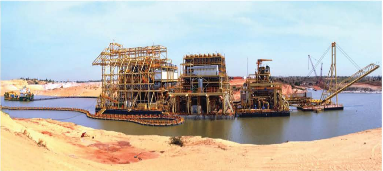
Dredge and Wet Concentrator Plant (WCP)
