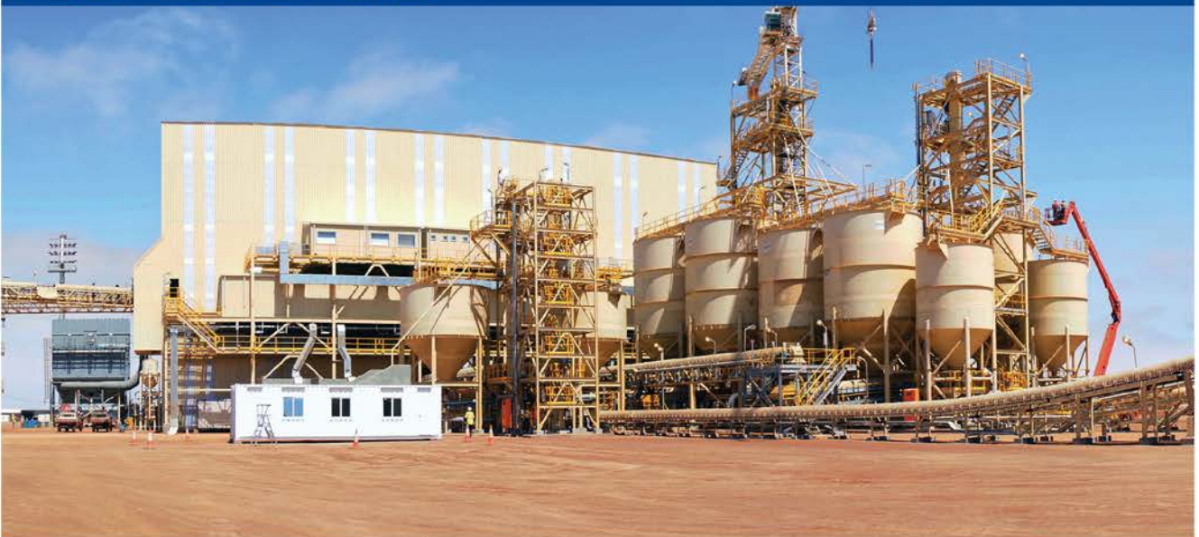
Dry Mill at the Mineral Separation Plant (MSP) with zircon and rutile storage
