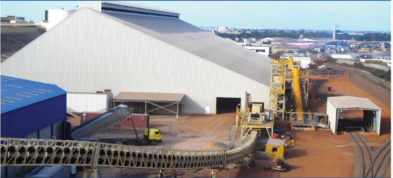
Storage and conveyor facilities at Dakar port
