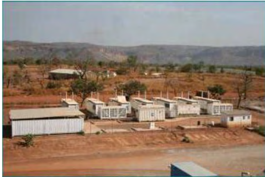
Figure 18-2 Tabakoto Power Plant
