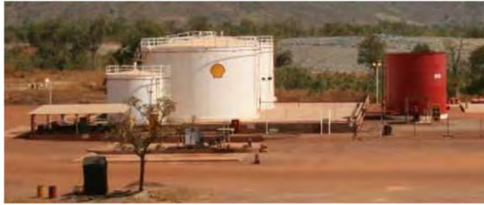
Figure 18-5 Diesel Fuel Storage
