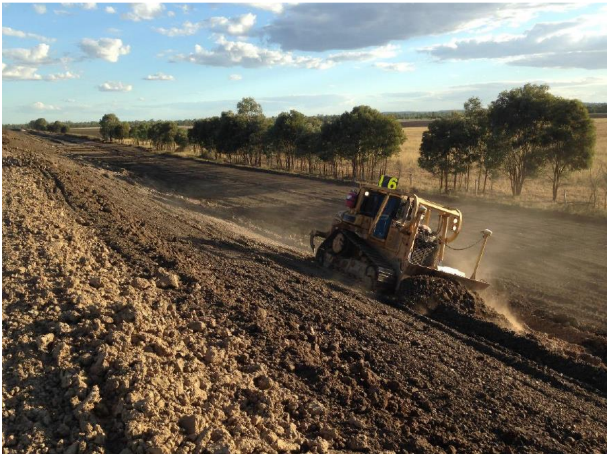
Figure 2 – Baralaba North Mine Western Levee Construction
