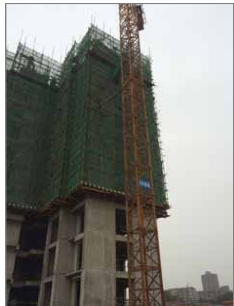
First residential tower under construction
