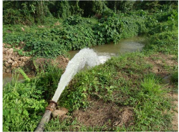
Removing water from mine pit continuously.
