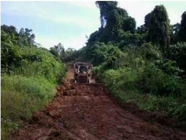
Tractor smoothing 1.2km of mining road from concrete road to mine.
