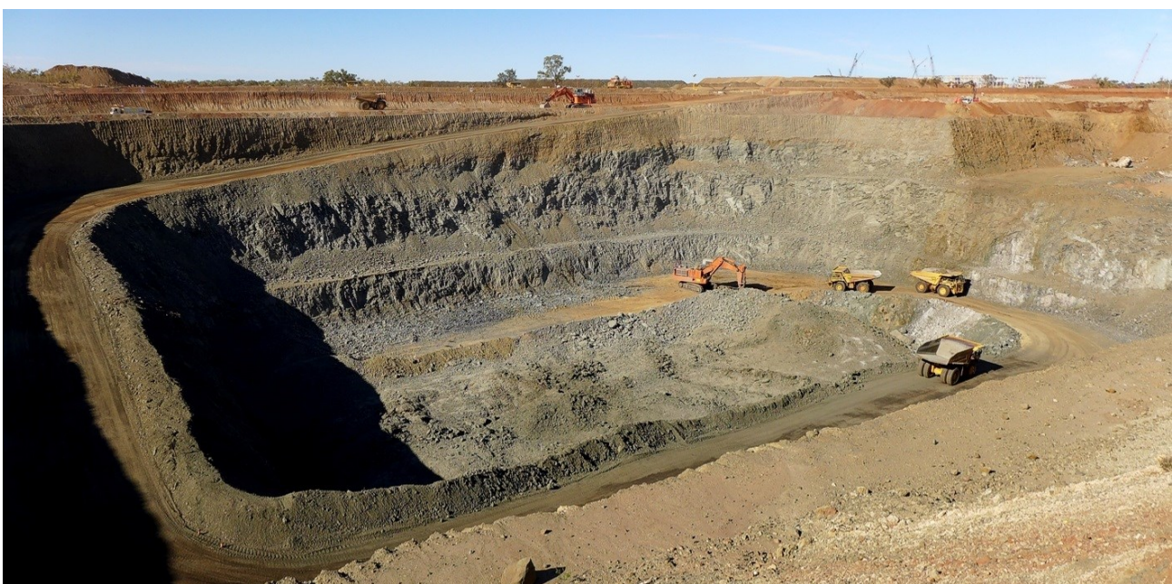
Figure 6: Top image shows current dig-plan schematic with current dig areas in yellow outline and drill areas in red outline. Below image shows the pit shortly after blasting of the ore zone on the floor of the pit. The waste area beside the ore will be removed first, leaving the ore proud for ore-mark-up and then selective mining.
