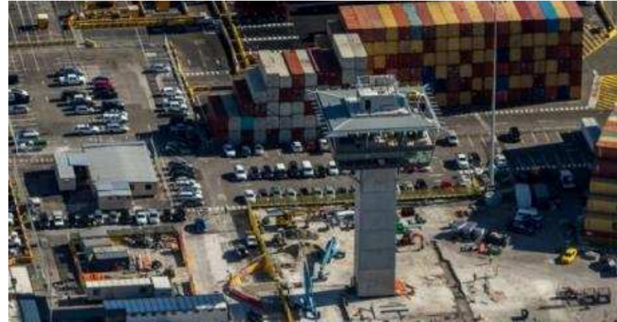
Admin Building Site as at May '14
