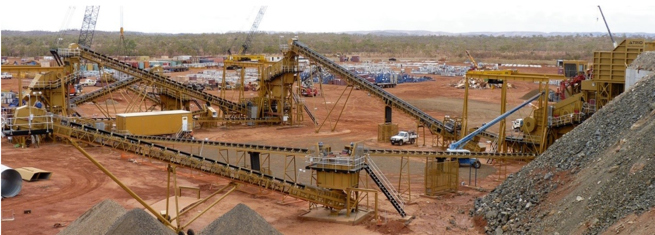
Figure 7: Crushing Circuit in foreground and numerous deliveries of steelwork and other componentry in the lay-down area in the background
