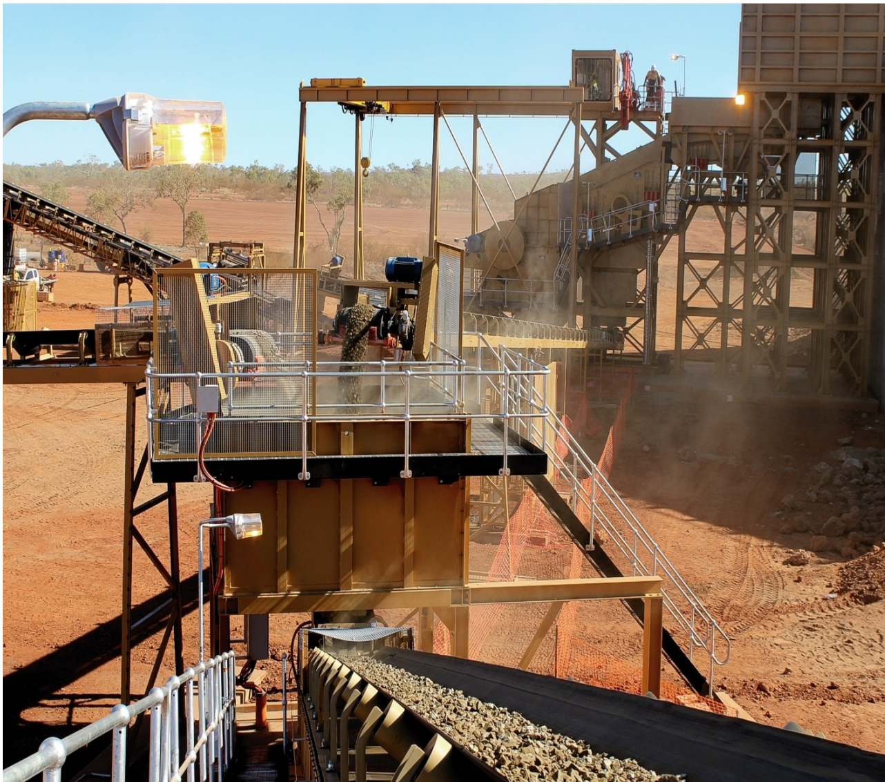
Figure 8: The Rocklands Crushing Circuit during test-crushing. Final product conveyor that will provide feed (-40mm) to the HPGR.
