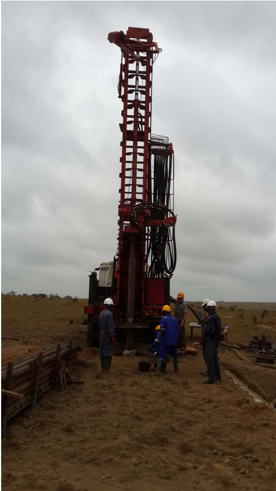
Figure 2. Drilling rig at ED_02
