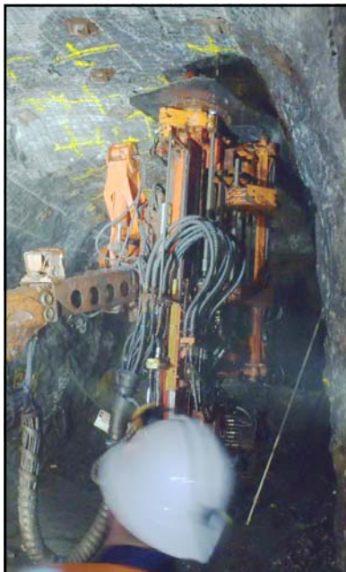
Underground drilling, Challenger
