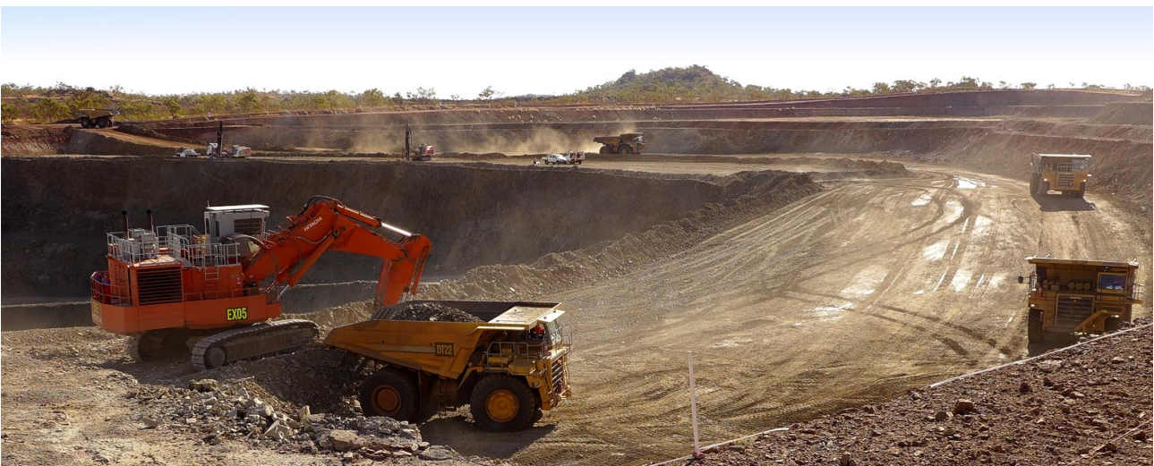
Figure 2: Mining on the shoulder of the LM2 Pit; LM1 Pit left background
