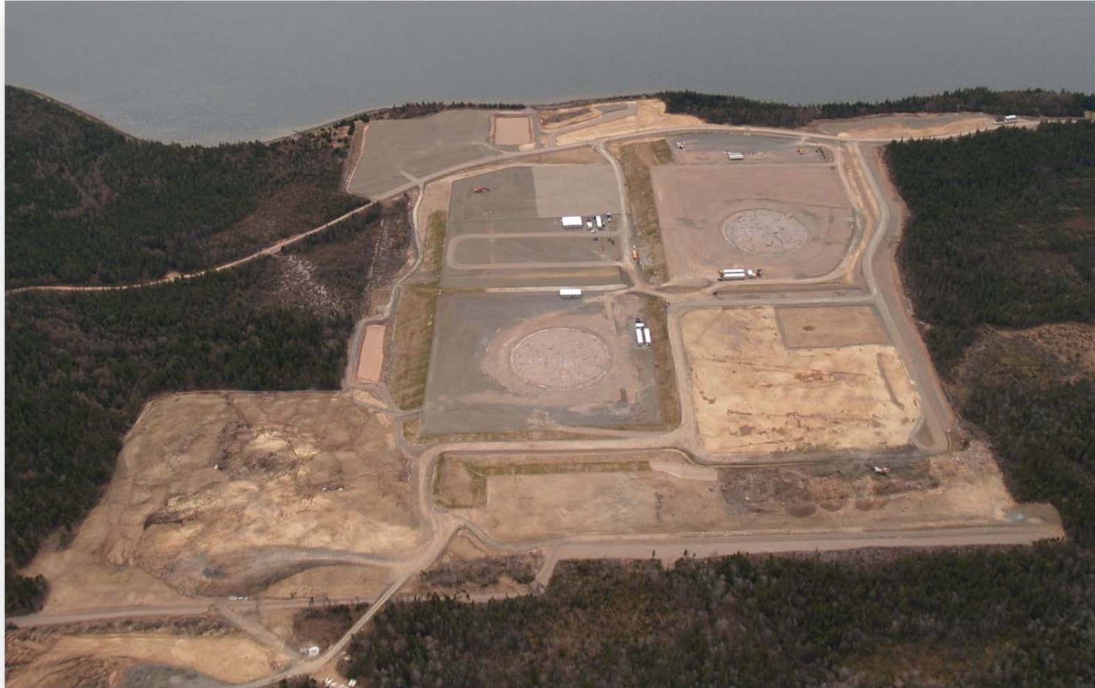
Figure 2: Aerial View of the Bear Head LNG Project Site, Nova Scotia, Canada
