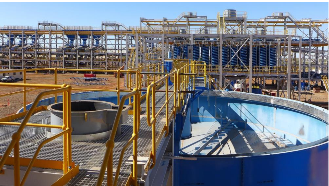
Figure 21: Top image shows Scrubber Circuit and bottom image shows the Gravity Jig building (far background), Spirals (middle distance) and copper concentrate thickener tank as viewed from the Thickener/Filtration circuit (foreground).
