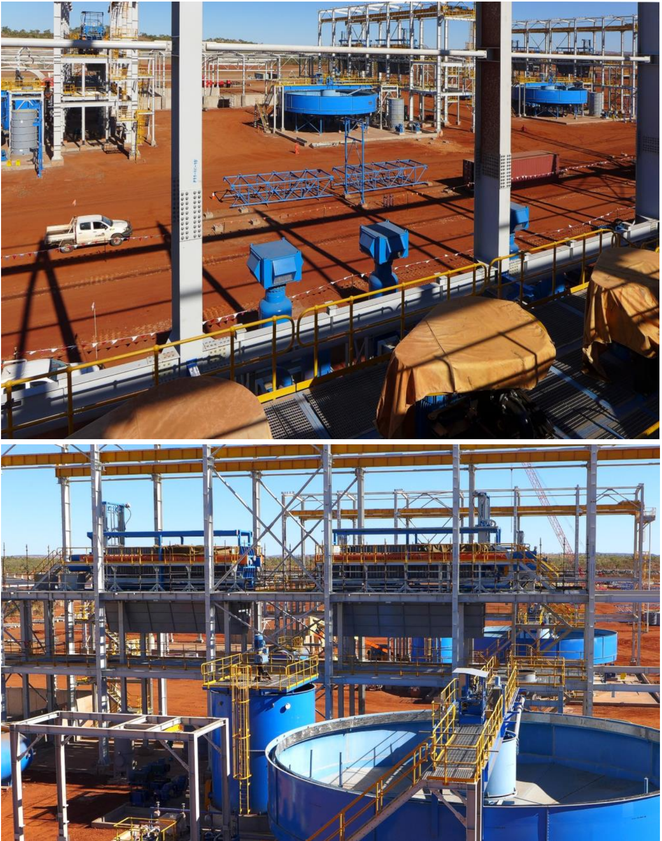
Figure 20: Thickener/Filtration circuits viewed from the Flotation Cell building (top image) and; Thickener/Filtration circuit up close.
