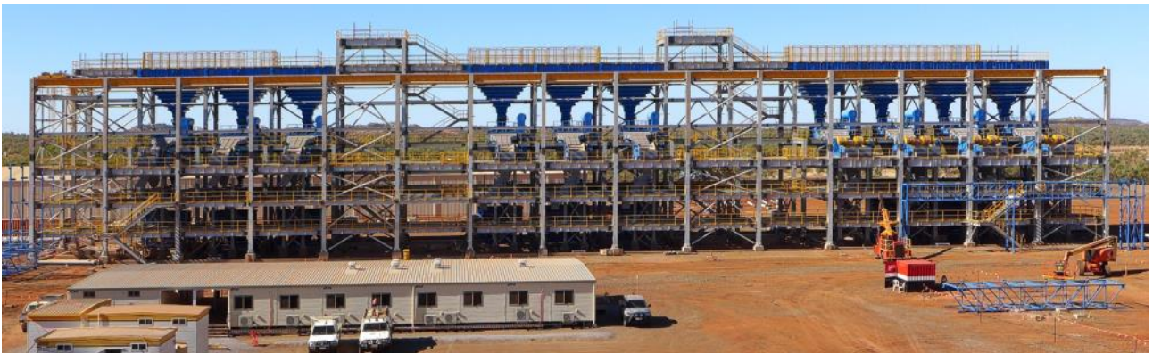
Figure 9: Rocklands Gravity Jig Circuit with multiple continuous gravity jiggging units (alljigs®) supplied by German Company allmineral, capable of recovering various native copper fraction sizes (see flow-sheet diagrams from page 61)
