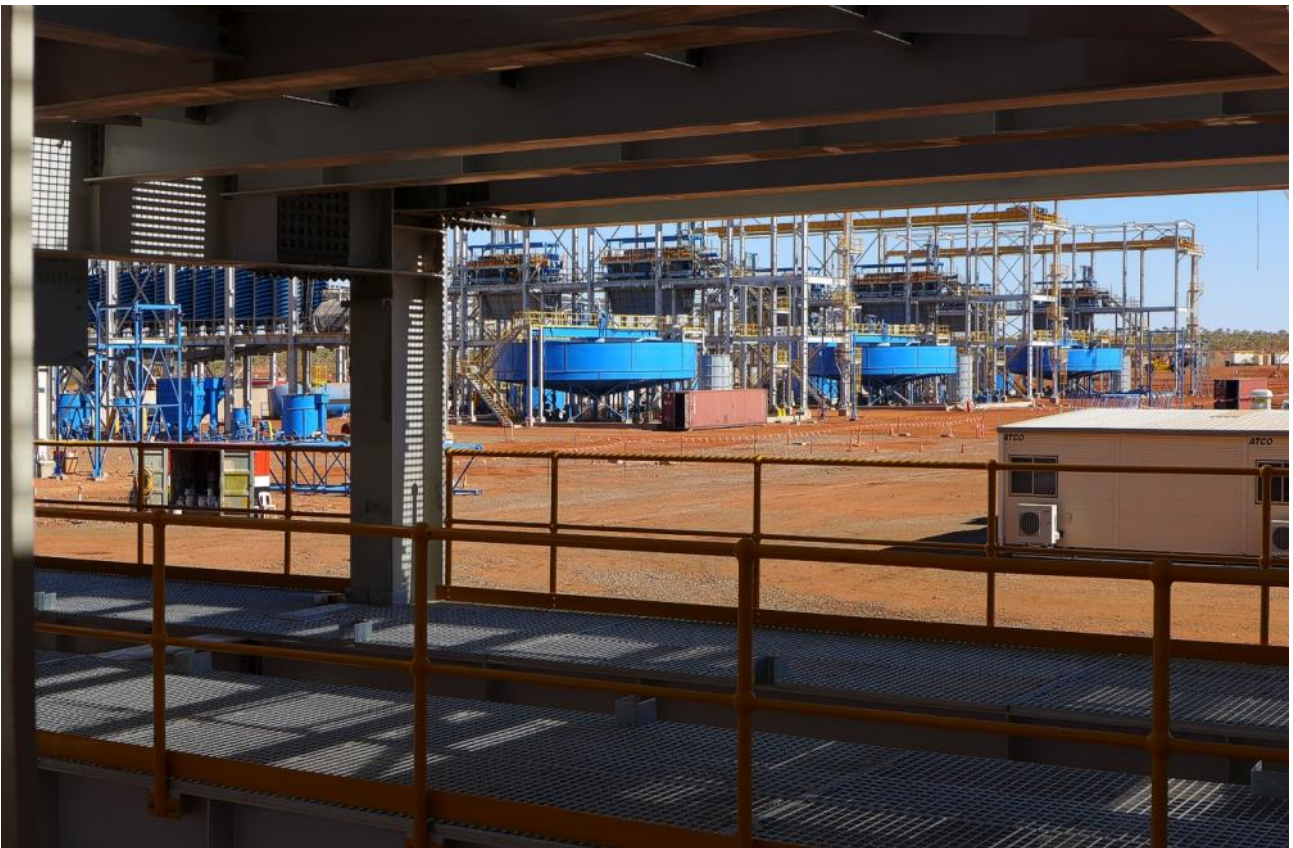
Figure 15: Flotation Cells (top image) and in background; Spirals (left) and Thickener/Filtration circuits (right three structures)
