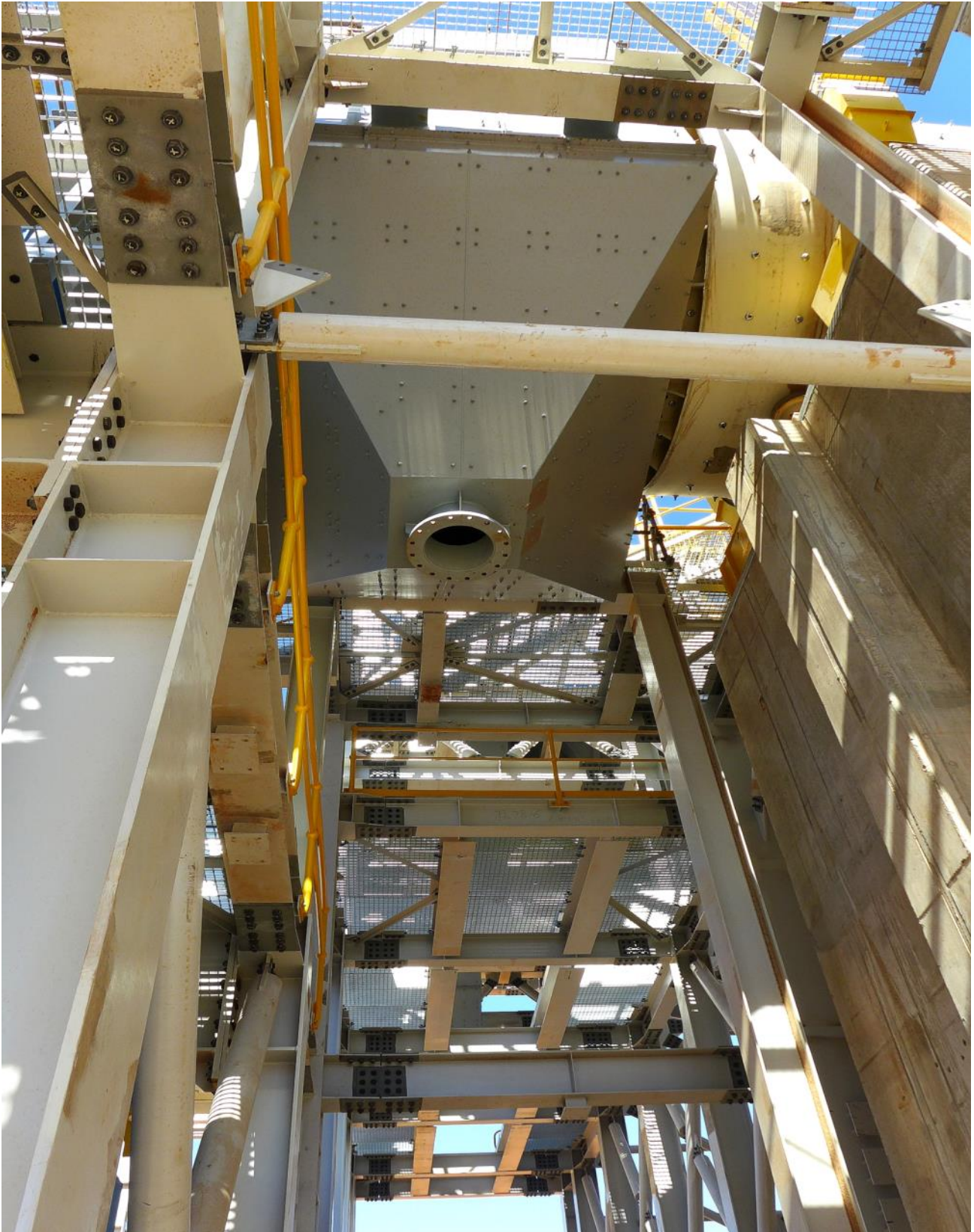
Figure 23: Scrubber discharge sump
