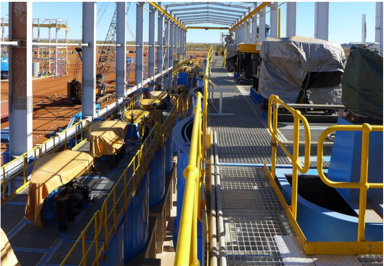
Figure 14: Flotation Cell building - flotation cells (top) and cell agitators (bottom)
