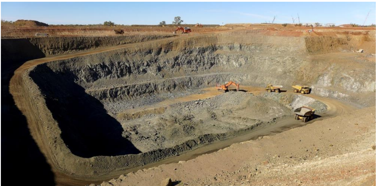
Figure 33: Top image shows current dig-plan schematic at mid June, with dig areas in yellow outline and drill areas in red outline. Below image shows the pit shortly after blasting of the RL170m ore zone on the floor of the pit. The waste area beside the ore (where the digger is) was removed first, leaving the ore proud for ore-mark-up and then selective mining,
