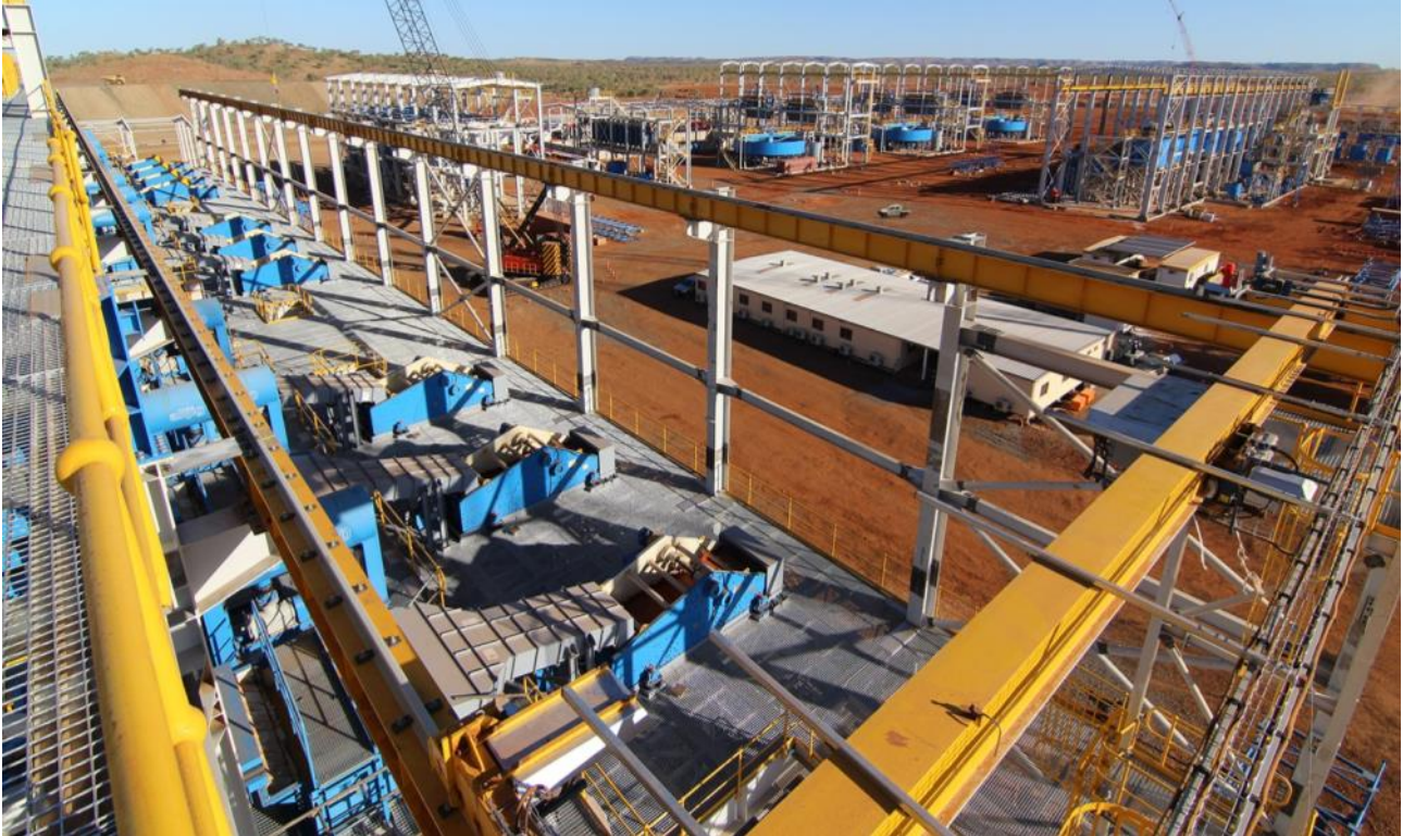
Figure 12: Gravity Jig Building - looking east; continuous alljig® units fade into the distance on level 3. From left to right in background; Table Separator Circuit; Spiral Separator Circuit; bank of three Thickener/Filtration Circuits; Flotation Cells; Cobalt Re-grind Circuit and; Magnetic Separation Circuit.
