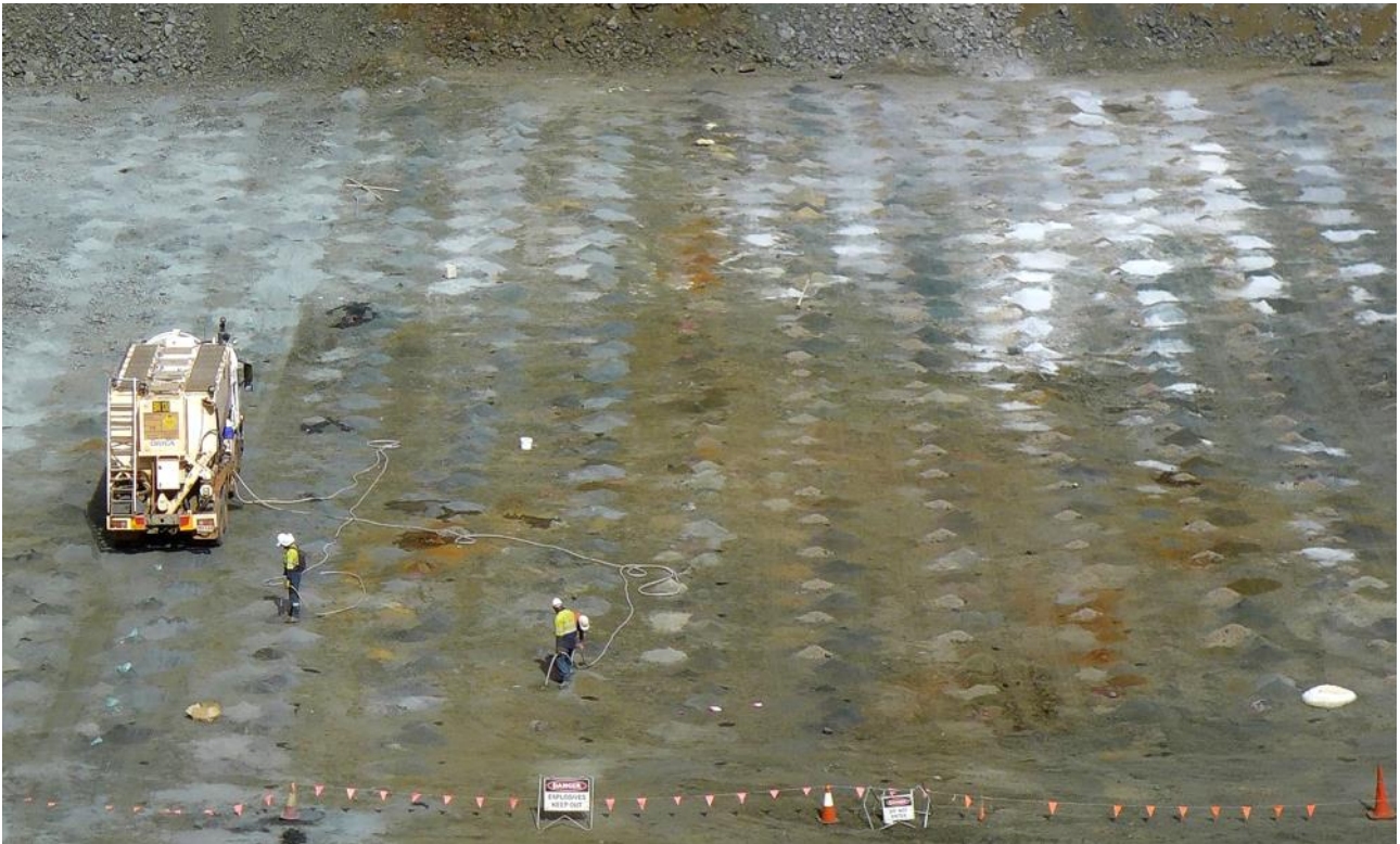
Figure 57: Blast-holes are sampled, geologically logged and sent for assay prior to being loaded for blasting. The changes in colour represent the different ore types, from primary with native copper associated (white colour), transitional chalcocite-rich native copper ore (black/grey), and high-grade supergene native copper ore in clays (olive/yellow/grey).
