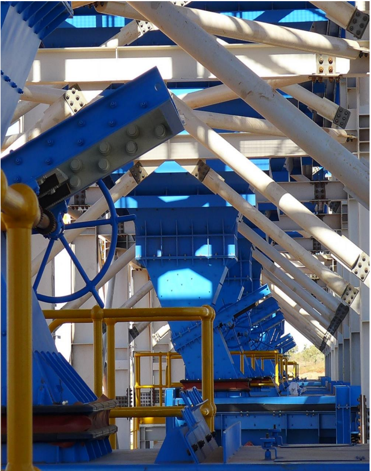
Figure 24: Gravity Jig Building - level 2 Jig-feed chutes and bank of continuous alljig® units.
