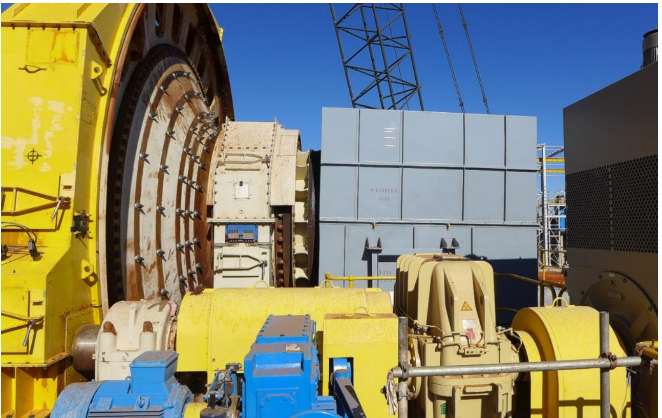
Figure 17: Ball Mill feed chute (above) and drive-train and trommel screen unit (grey box - centre)
