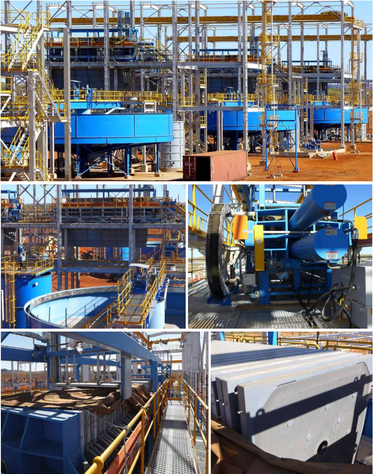
Figure 22: Thickener/Filtration circuits (above) and close up of filtration unit and panels (bottom images)
