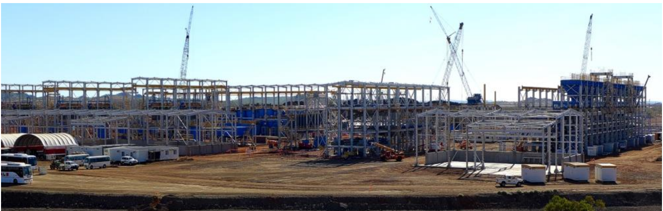
Figure 10: Rocklands Process Plant - major components installed, structural completion underway.
