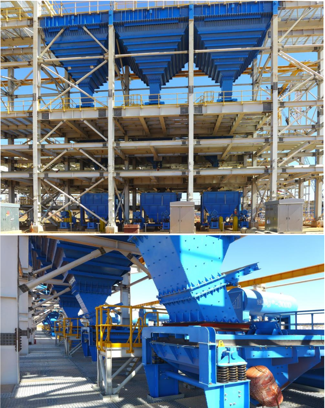
Figure 3: Gravity Jig Building - Top image; feed bins (top), screen on middle floors and pump-boxes on ground floor. Feed chutes into ore jigs.
