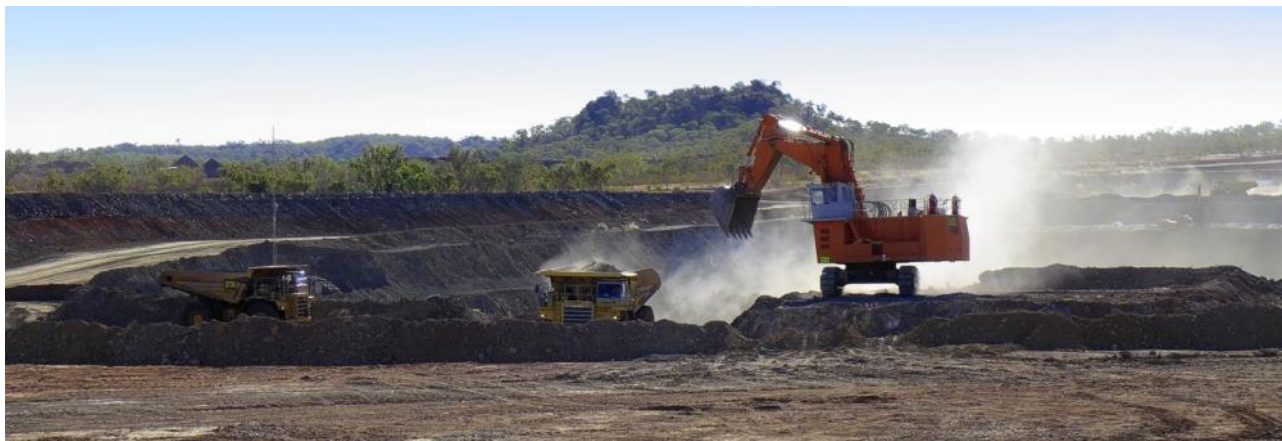
Figure 41: Stage-2 (LM2) pit has commenced, whilst the deeper LM1 Pit (behind the excavator) continues to be deepened.
