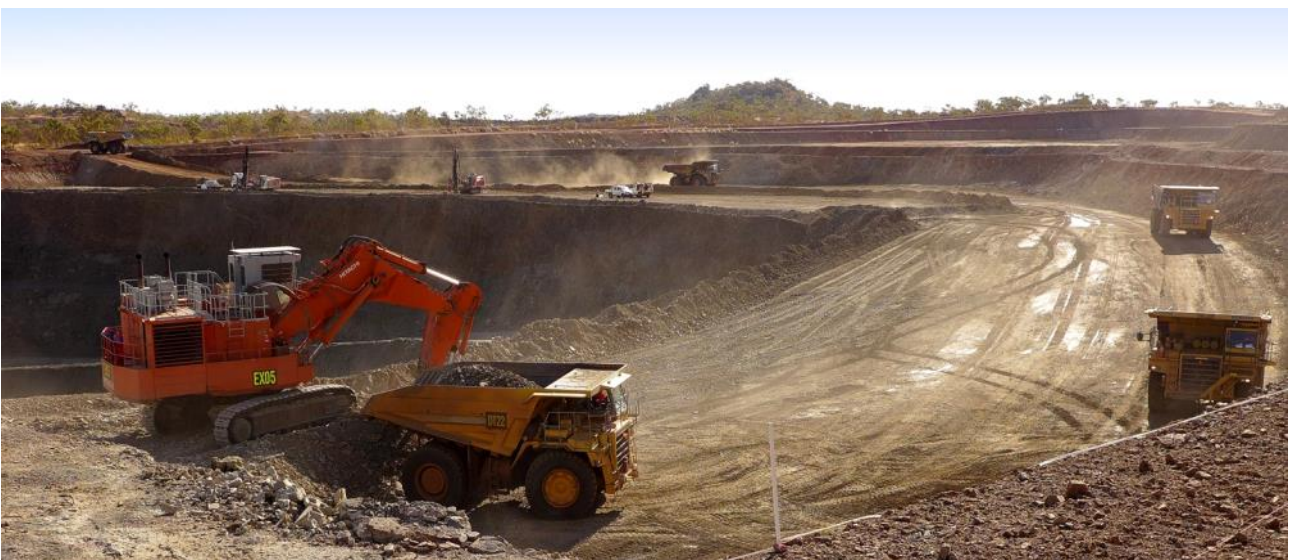
Figure 5: Mining on the shoulder of the LM2 Pit; LM1 Pit left background
