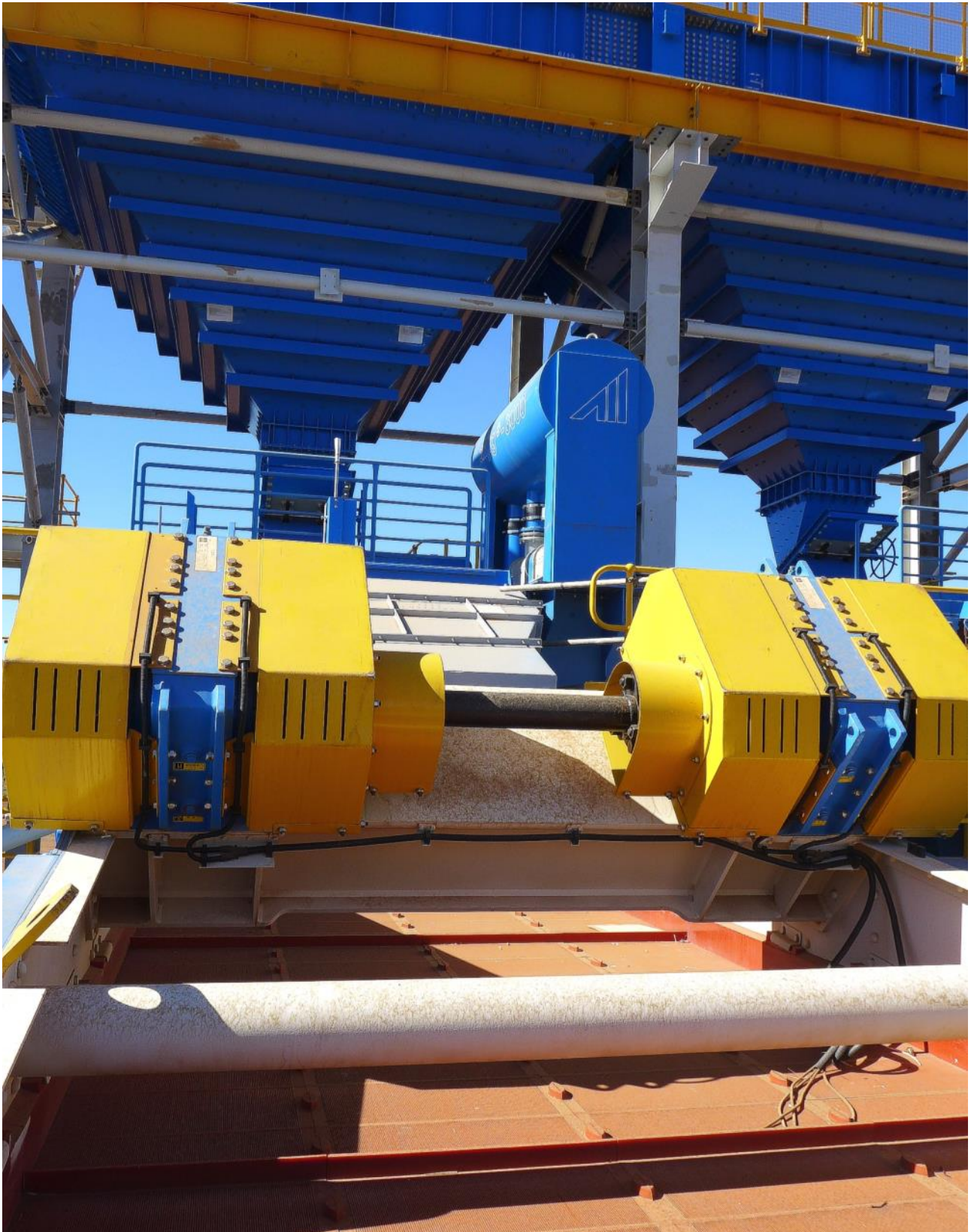
Figure 16: Gravity Jig Building - feed bins (above) and close-up of lights screen (foreground).
