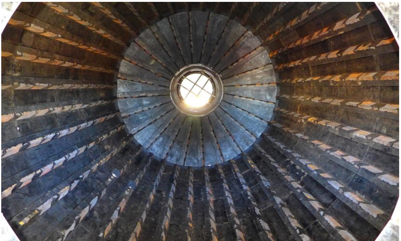
Figure 19: Ball Mill discharge trommel (top image) and high-impact poly-met lining of Ball Mill almost complete (bottom image)
