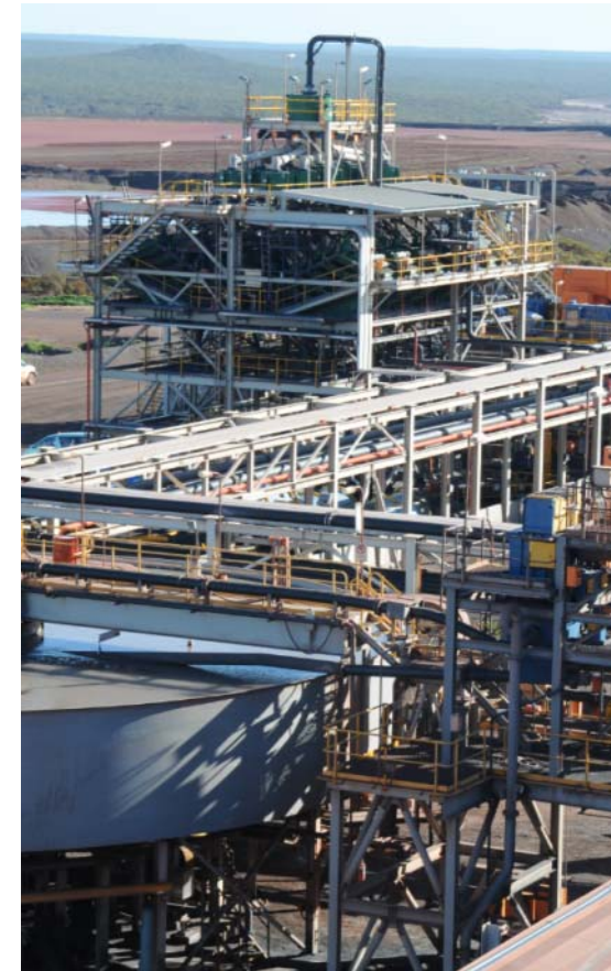
Magnetite Expansion Project, South Middleback Ranges, SA
