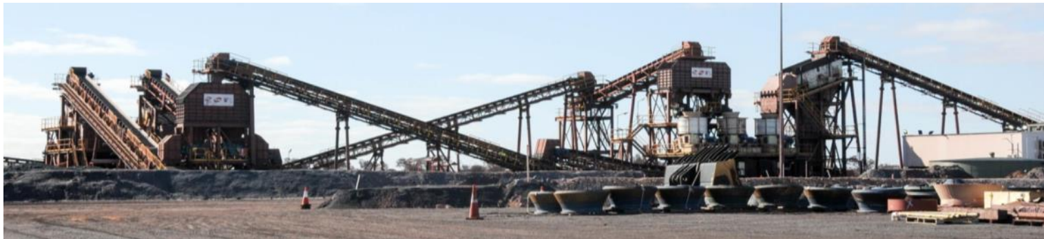
Wirrida Crushing & Screening, Southern Iron, SA
