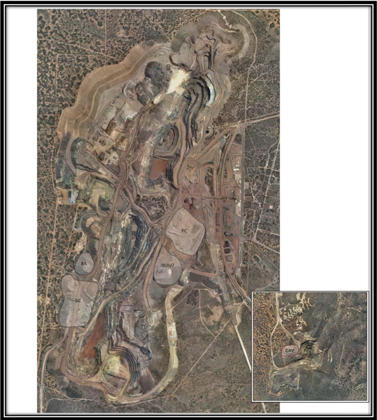
Figure A2: Iron Baron LGO Stockpile Locations
