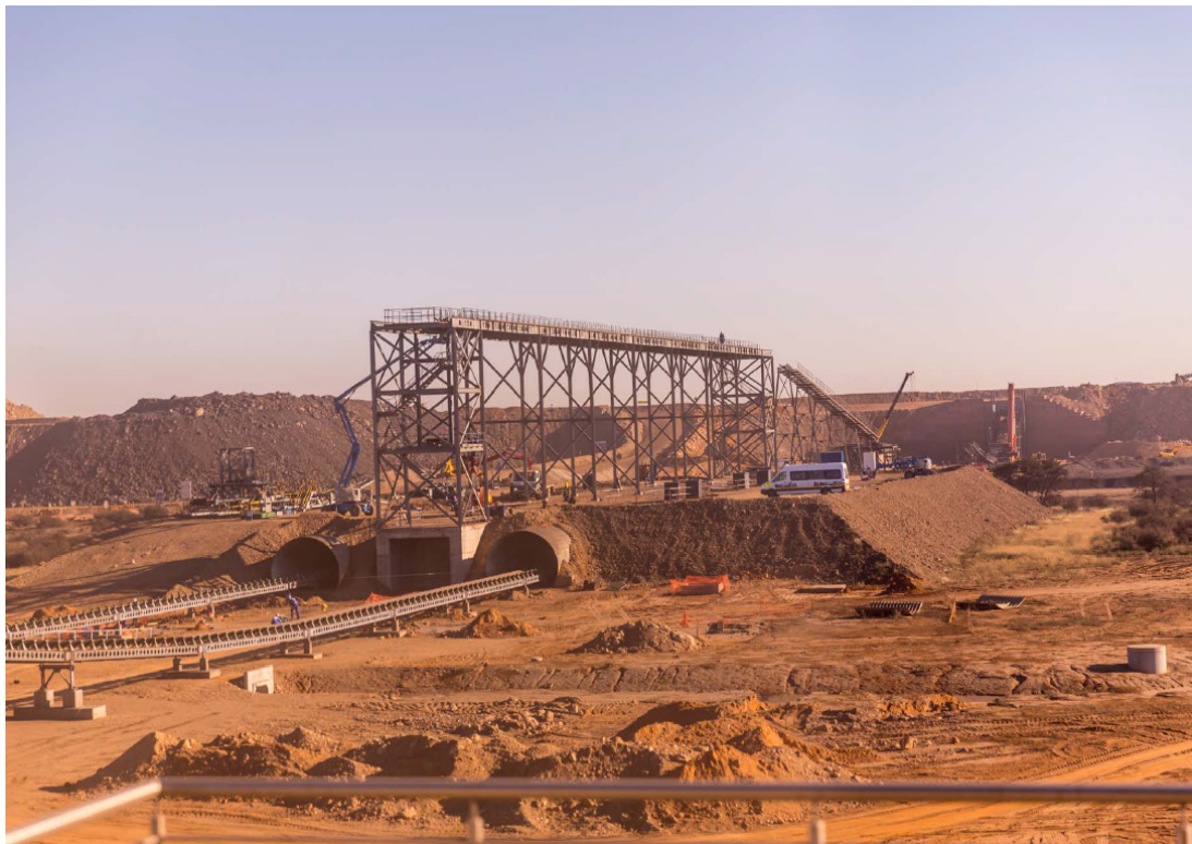
Crushing and screening plant under construction
