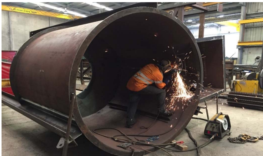
Beneficiation plant pump hoppers being fabricated in Perth during the quarter
