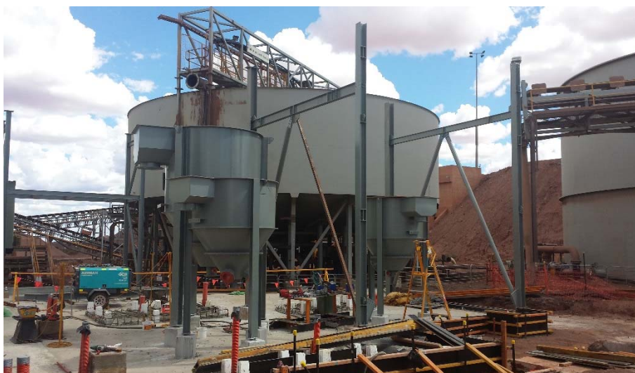
Beneficiation plant foundation and structural work at Windimurra
