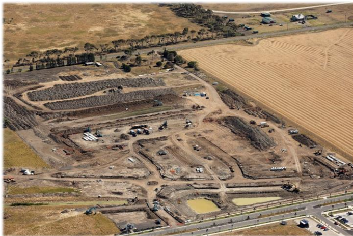
Wetlands and Stages 2, 3 and 4 in progress
