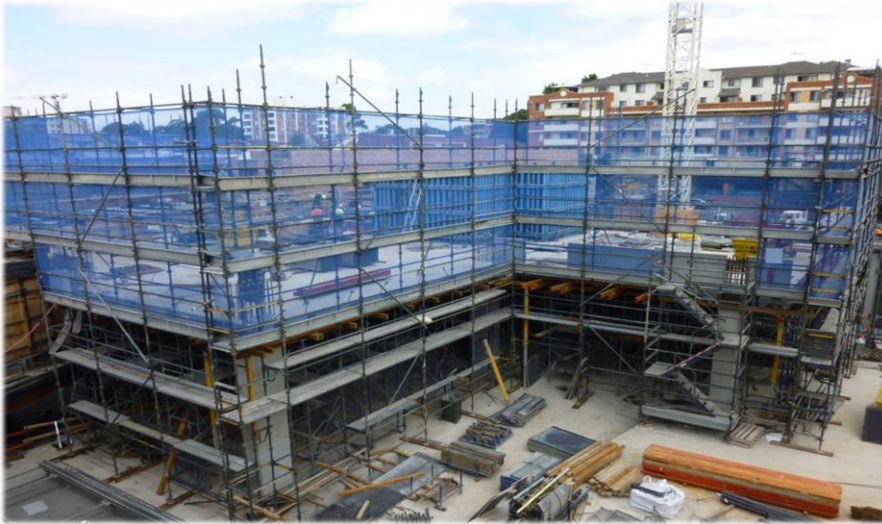
Preparing L3 Formwork Building B
