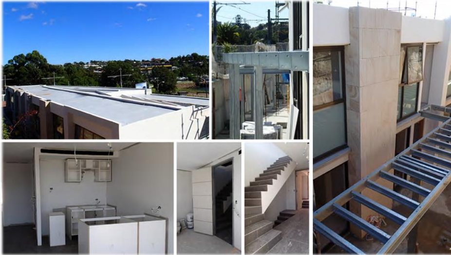
Block A-E structure complete
