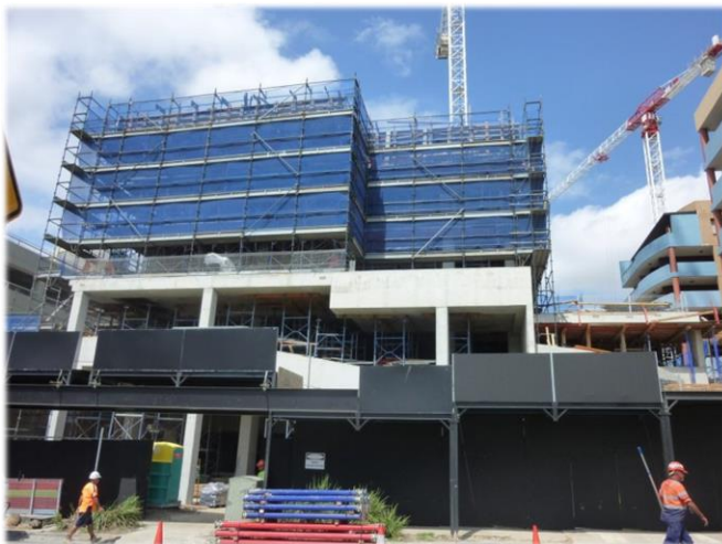
Wynne Avenue Scaffolding stripped
