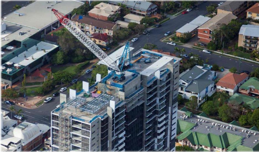
Roof structural steel underway
