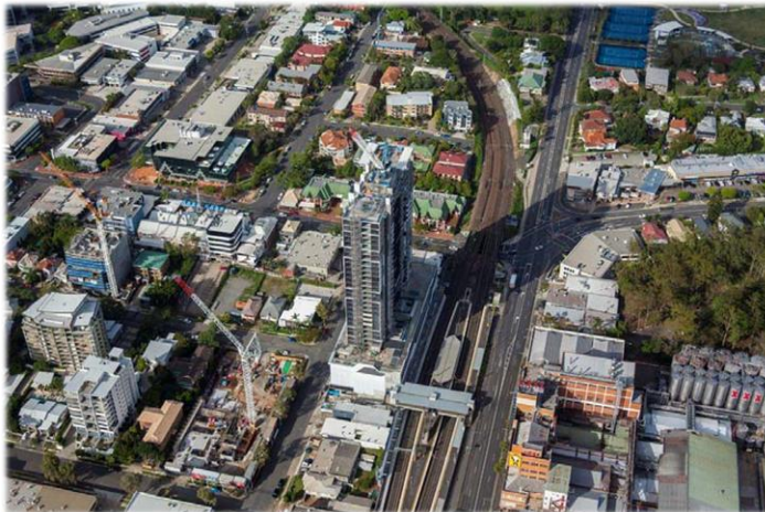
Eastern side of building
