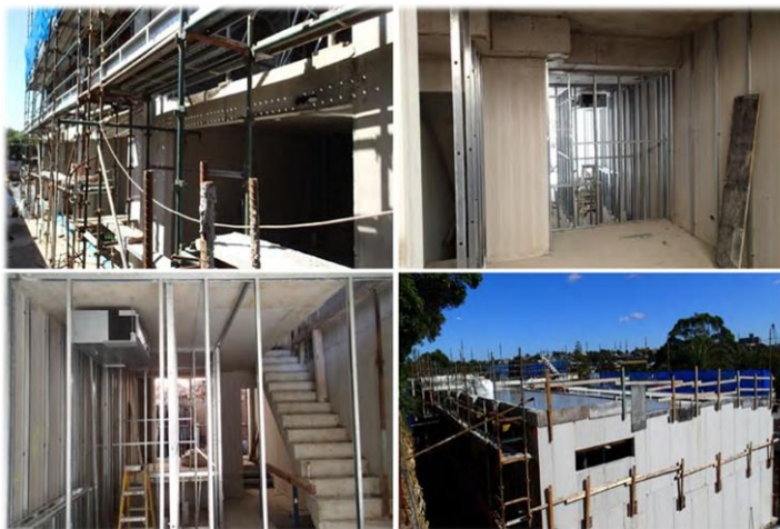
Mechanical, hydraulic, electrical in working progress
