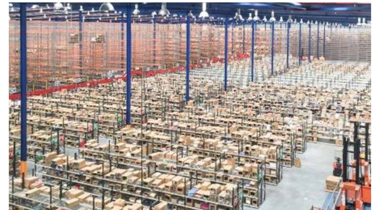
New Australian National Distribution Centre
