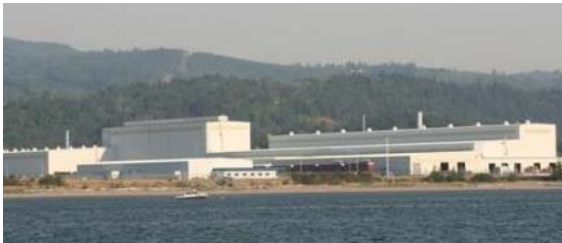
Metal coating & painting facility, Kalama, WA
