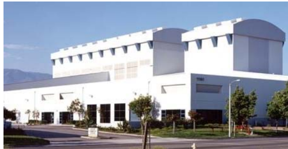
Metal coating & painting facility, Rancho Cucamonga, CA
