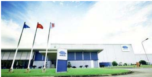
Metal coating & painting facility, Phu My
