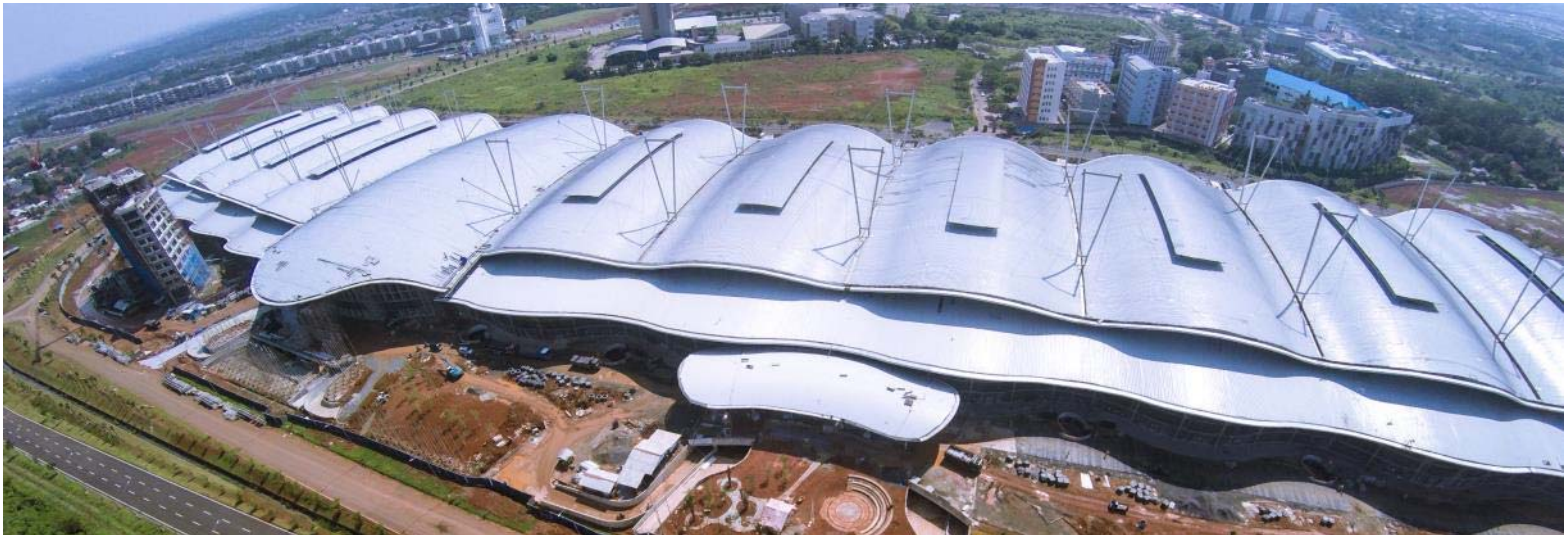
Indonesia International Expo Centre – biggest convention hall in ASEAN
