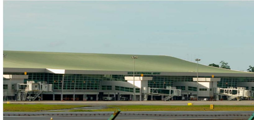
Kuching International Airport, Sarawak
