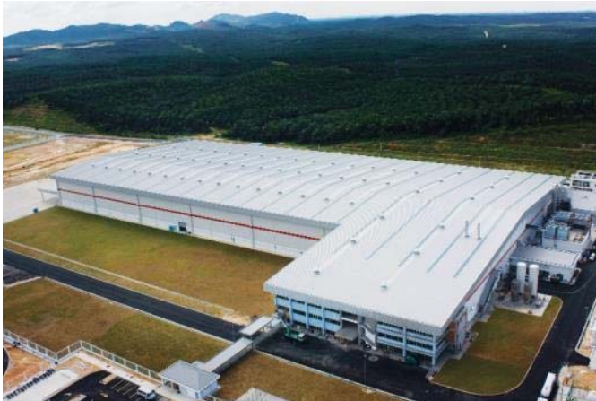
Coca-Cola Bottling Plant
