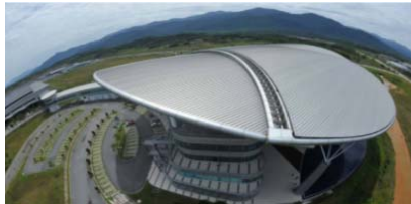
Proton City Admin Building
