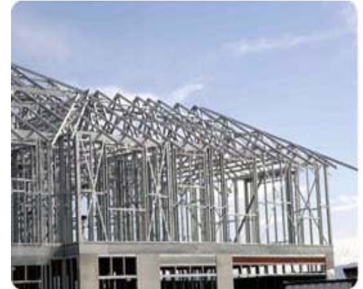
Framing and truss
