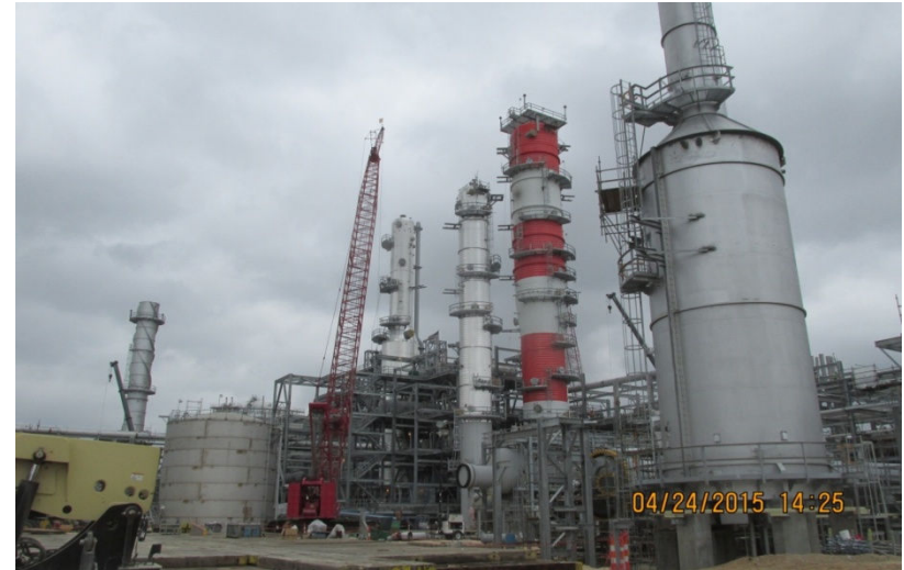
Heavy lift columns installed – CO2 absorber installed
