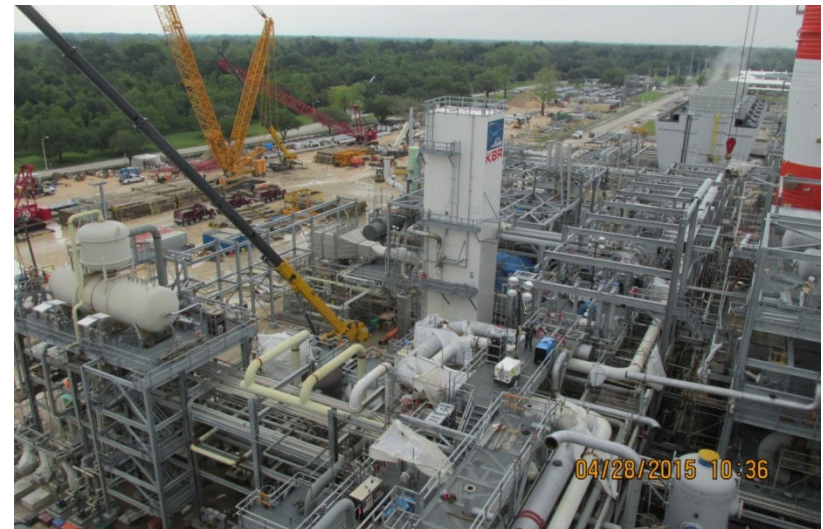
Overview looking south
