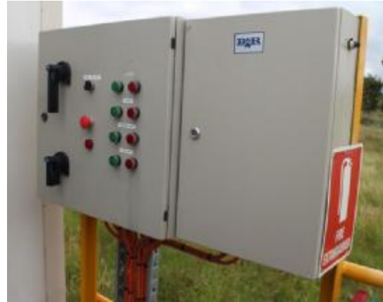
Gravity Plant MCC
