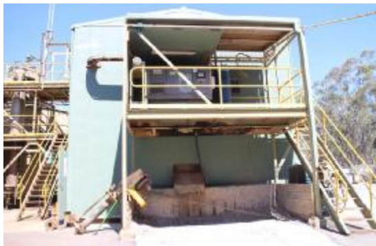
Mill Scats and Air Compressors
