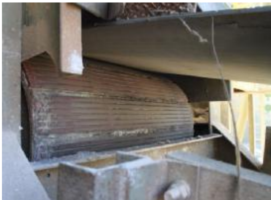
Head Drum of Reclaim Conveyor
