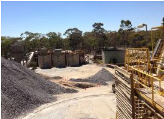
Leach, CIP and Water Tanks
