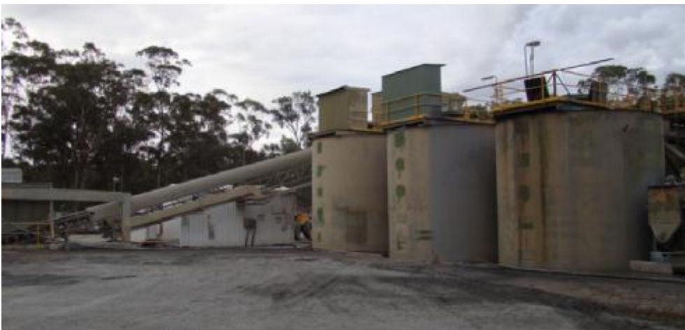
Porcupine Flat Gold Processing Plant, Maldon Victoria
