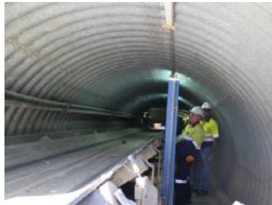
Reclaim Conveyor and Tunnel
