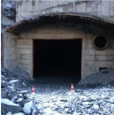
Existing entrance to Underground Mine Infrastructure at Bjørnevatn
