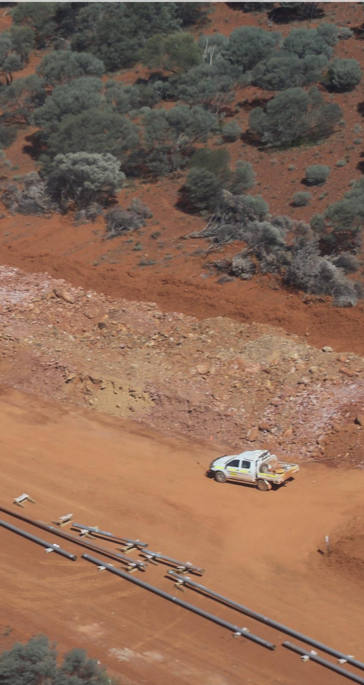
Construction of the new Eastern Goldfields Pipeline, WA is well underway with almost half of the 292 km of pipe strung along the route. Completion due by January 2016.
