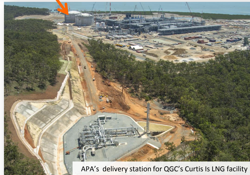
Connection point on QGC's Curtis Is LNG facility
