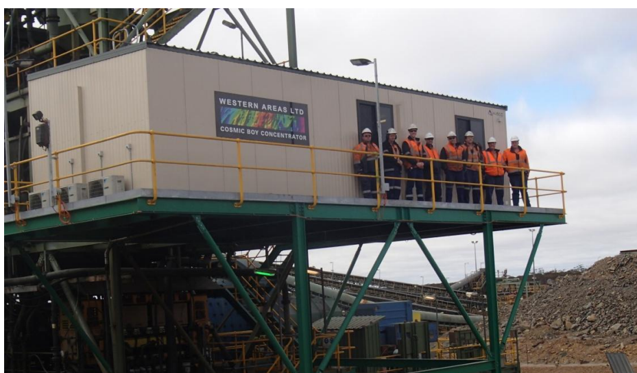
New Cosmic Boy Concentrator Control Room
