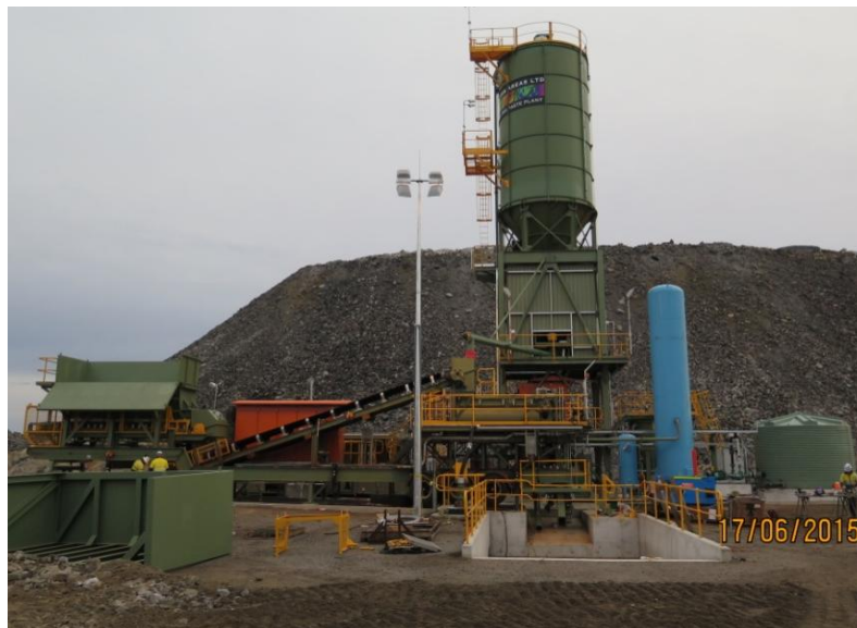
Commissioned Flying Fox Paste Fill Plant
