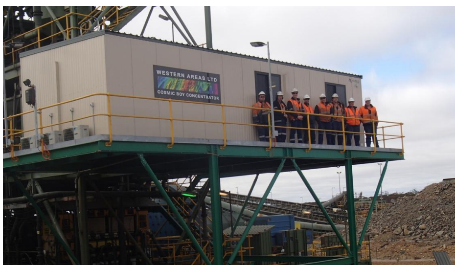
New Cosmic Boy Concentrator Control Room
