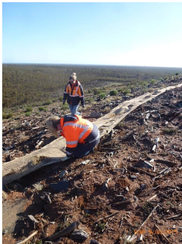
Environmental Technicians Lauren Curlewis and Louise Pearman undertaking erosion control work and seedling planting on the Spotted Quoll waste dump.
