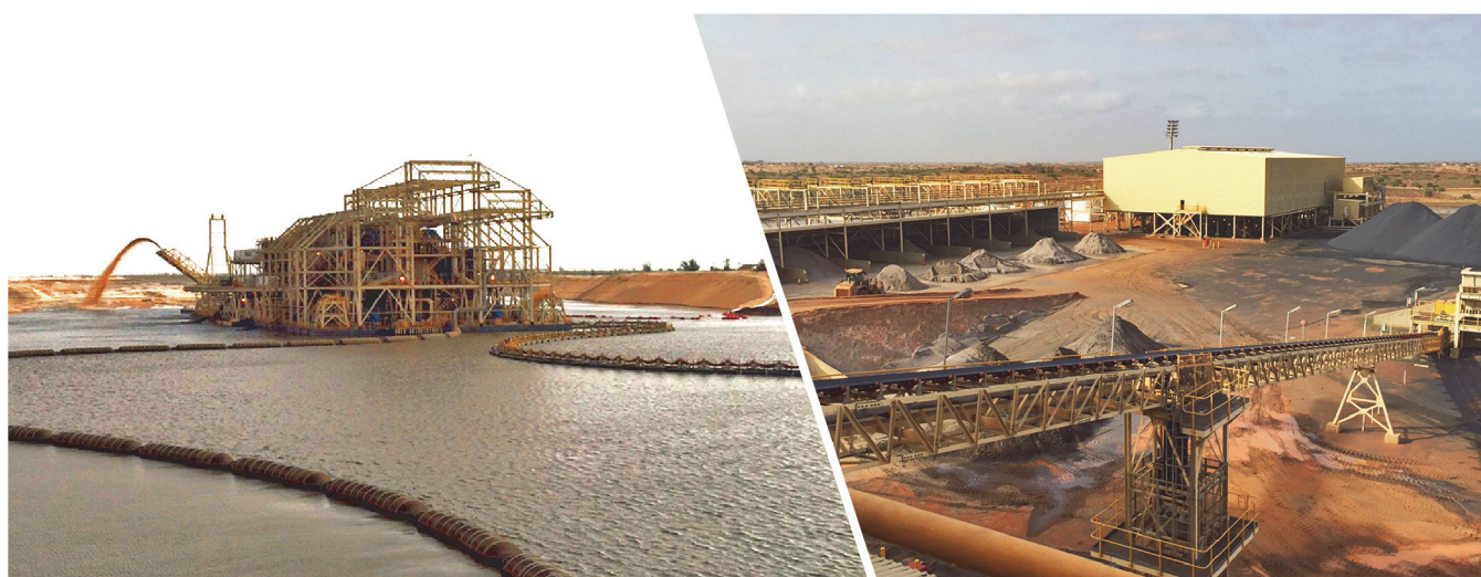
Grande Côte Operations Wet Concentrator Plant and Mineral Separation Plant
