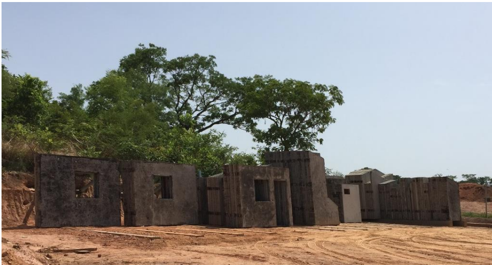
Picture 1: Banfora Gold Project | Locally Fabricated Panels for Resettlement Houses
