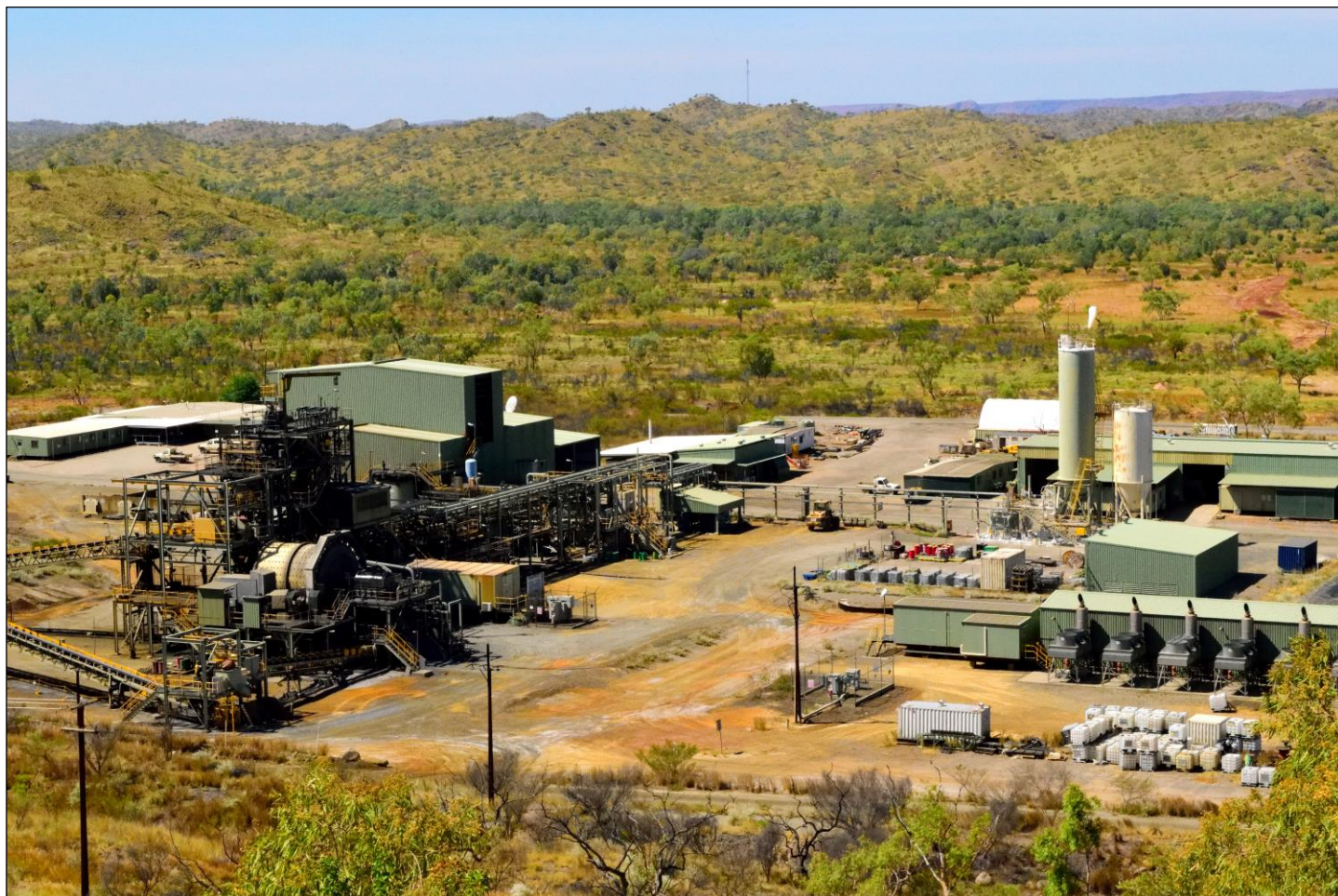
Photo 1 – Savannah Process Plant and Power Station
