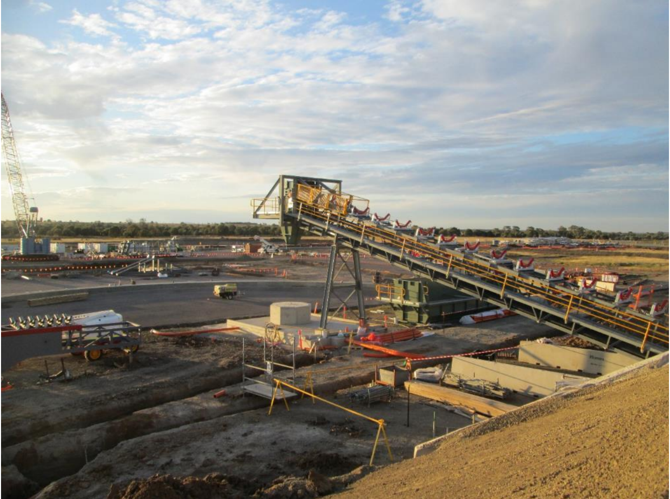
Figure 2 – Train Load Out Development In Progress
