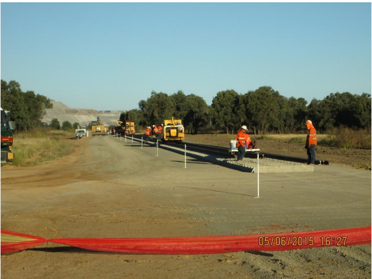
Figure 1 – New track laying to join Cockatoo’s new Train Load Out into the existing rail network.
