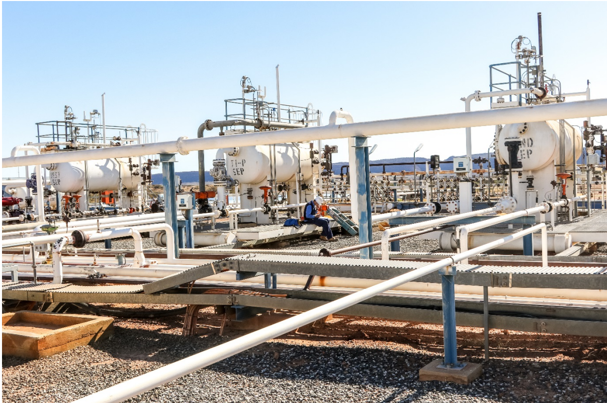
Figure 1: Merenie Oil & Gas Field: Eastern Satellite Station Oil and Gas Separation Equipment
