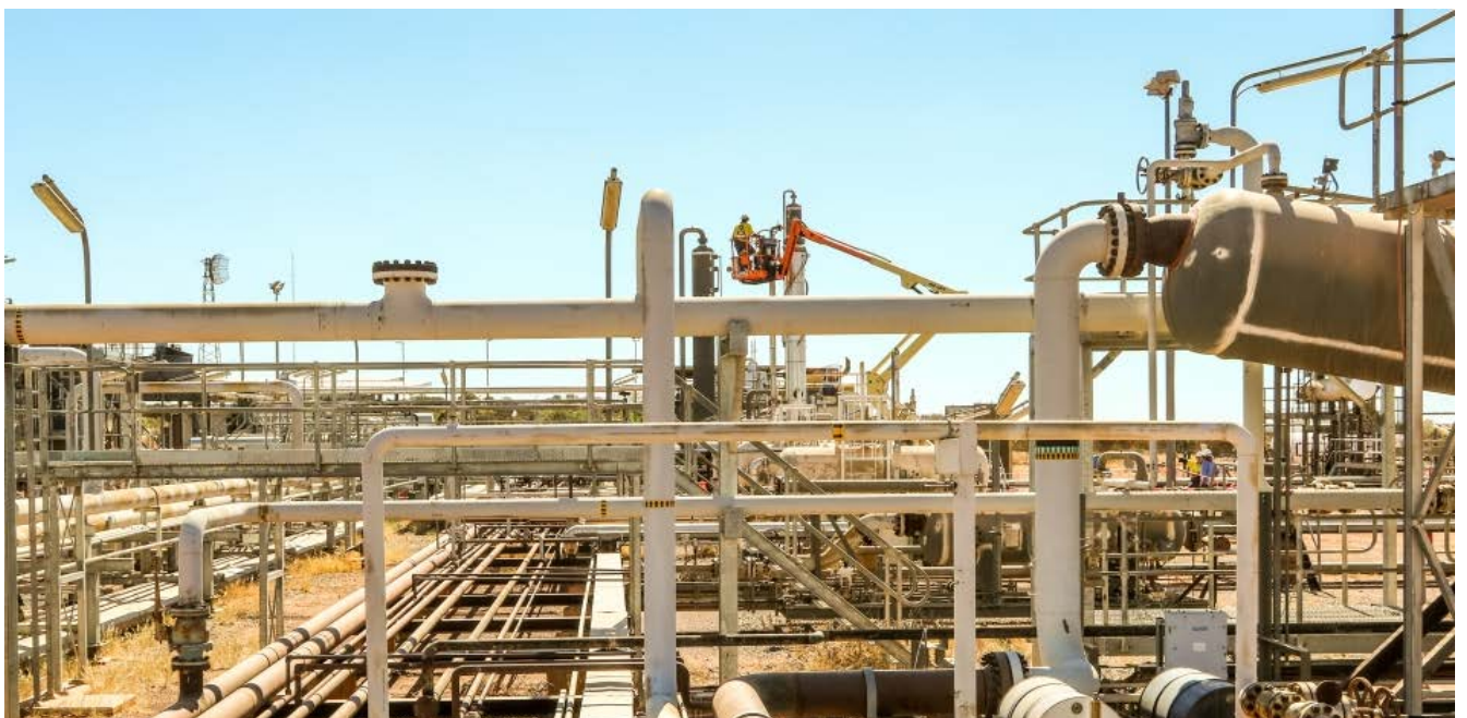
(Top left) Figure 5: Eastern Satellite Station Oil, Gas and Water Separator. (Top right) Figure 6: New 12" Flowline & Test skid. (Middle left) Figure 7: Central treating plant inlet separator free water knockout at CTP (Middle right) Figure 8: Eastern Satellite Station coalescing filter and plant pipeline rack. (Bottom) Figure 9: Central treating plant piping with maintenance work progressing.
