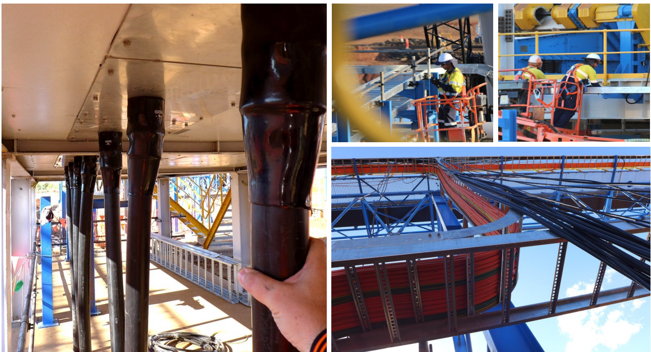
Figure 4: Electrical and computer cable installation is well underway at Rocklands and represents one of the largest, most important and complex contracts undertaken on the Project
