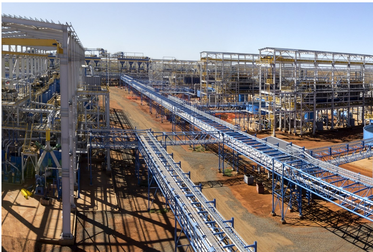
Figure 3: Flotation cell building (left), gravity jig and spirals building (far distance) and concentrate thickener & filter buildings (right) connected by a highway of piping and electrical cable support frames (foreground).
