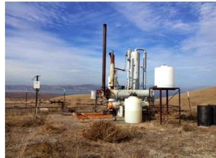
Los Medanos Production Facilities
